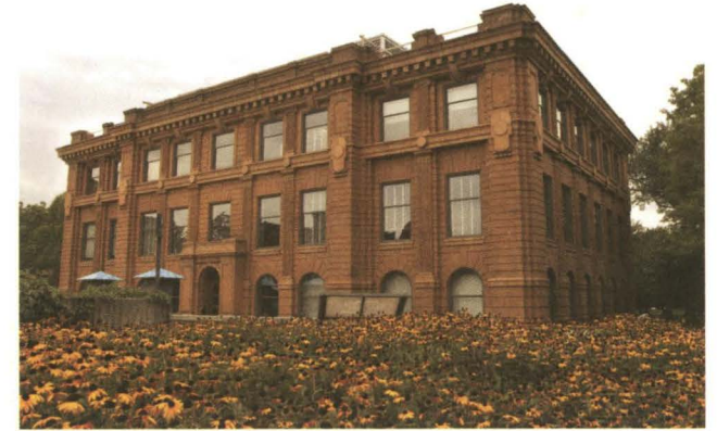
Jones Hall is a recent example of the University's investment in historic renovation and adaptive reuse.
