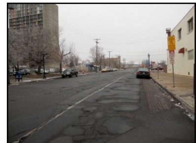
Figure 5: Potholes and uneven pavement on 4th
