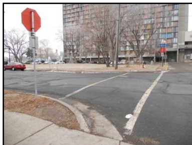
Figure 3: No access ramp at crosswalk on 15 th Ave.
