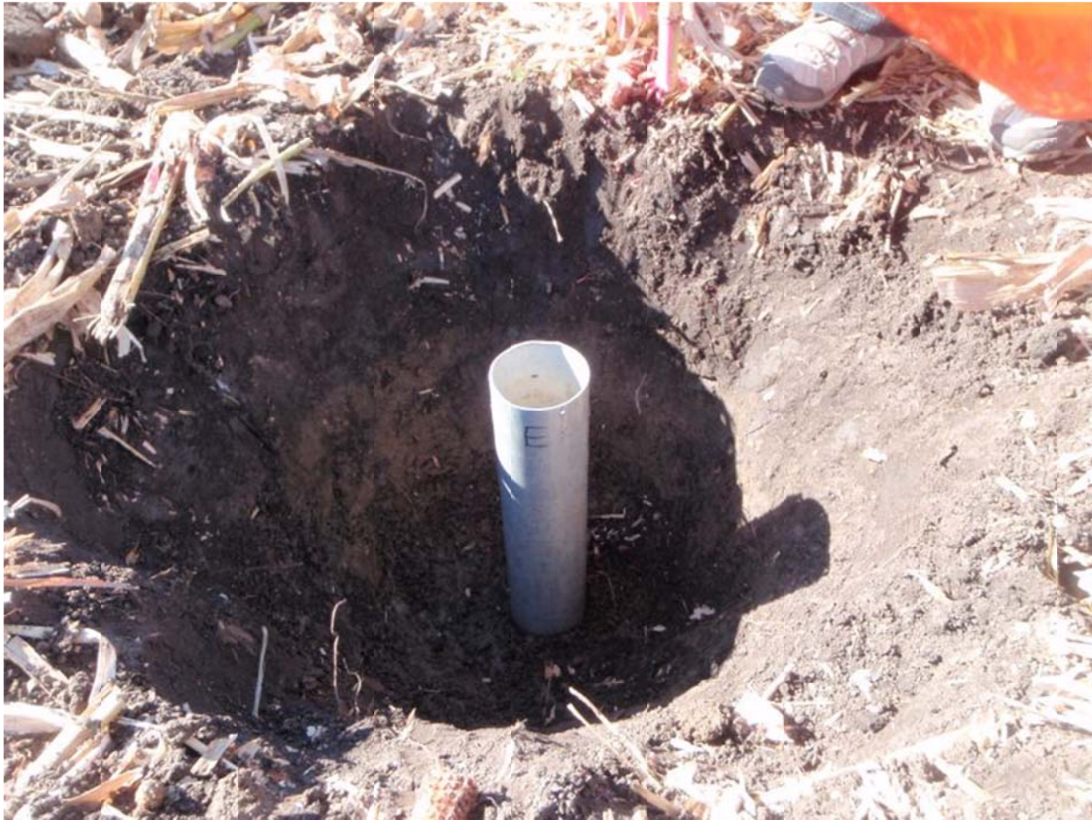
Figure 3.4 MPD installed in hand-dug hole
