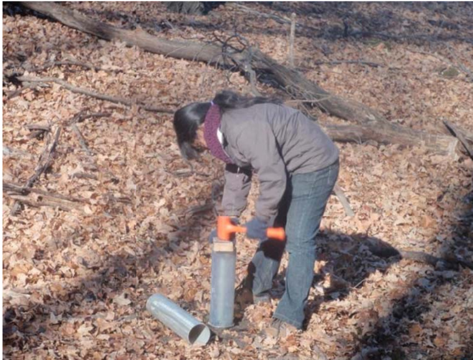
Figure 3.3 Installing the “new” MPD at the surface
