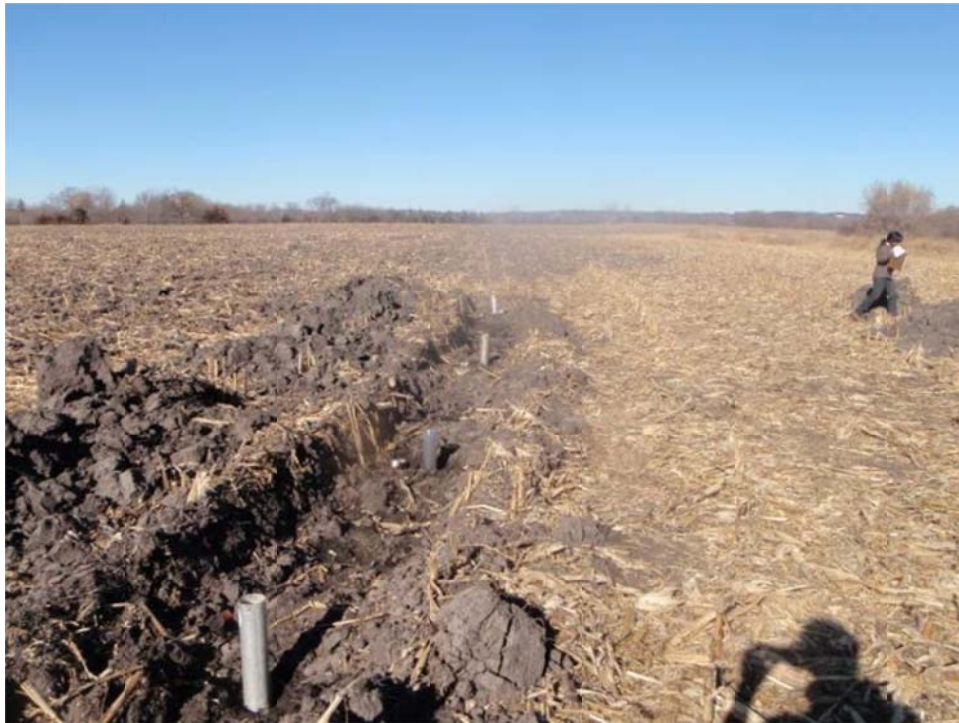
Figure 3.2 Trench dug by the excavator
