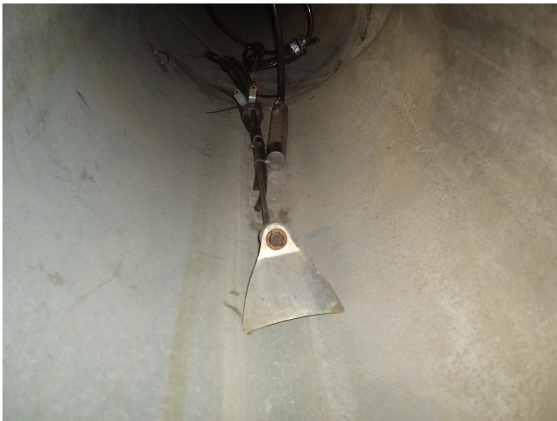
Figure 14. Strainer or manifold (right rear) and winged arm sampler (left front) installed in outfall
