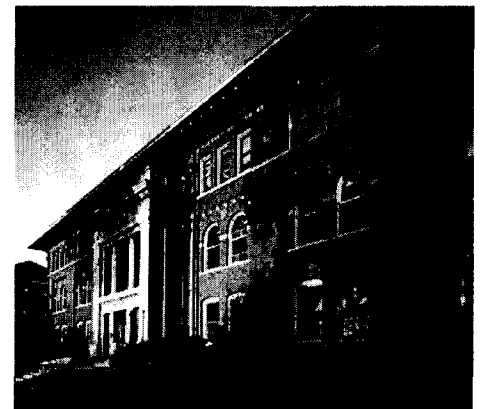
Biosystems and Agricultural Engineering building at UMTC in St. Paul
