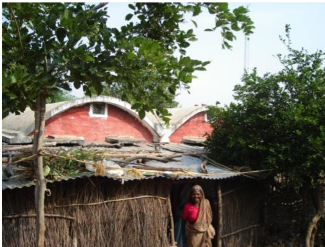
Figure 4.5: The CSV roofs as they appear in the Village of Waagdhara.
