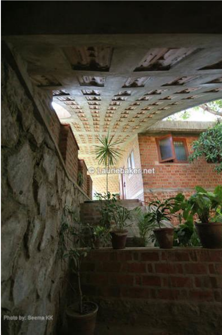
Figure 3.16: Laurie Baker. Self Employed Women's Association Building [Sewa Vilaapshala], photograph by Seema K.K., http://lauriebaker.net/work/work/pictures-of-buildings.html (accessed 03/16/2011).
