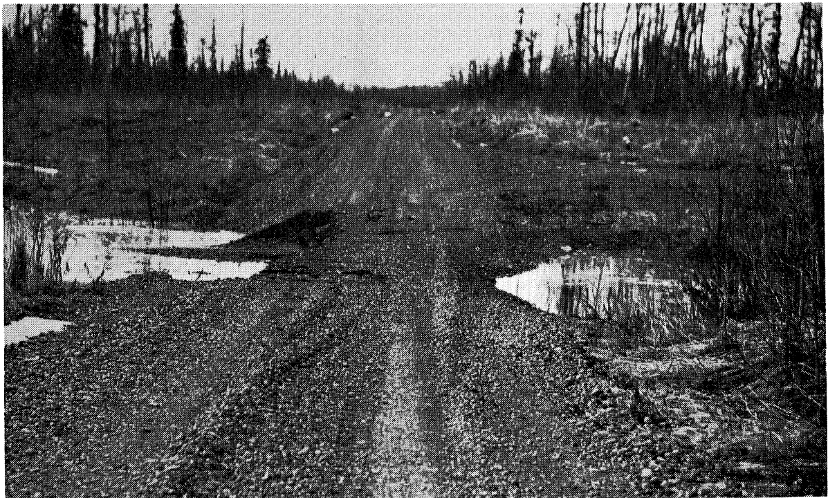
High river stages of May 16, 1948 created a discharge which exceeded the culvert capacity of this site.
