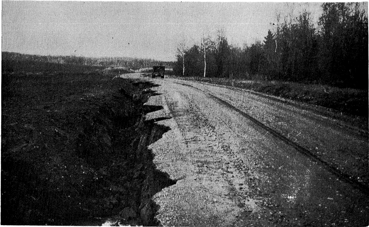
This gully resulted even though the ground was frozen.
