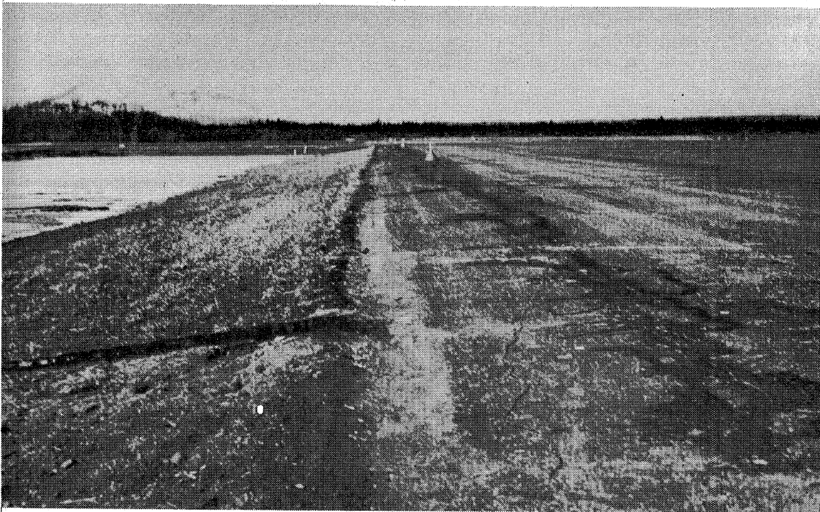
The drainage structure at this section is made of oil drums.
