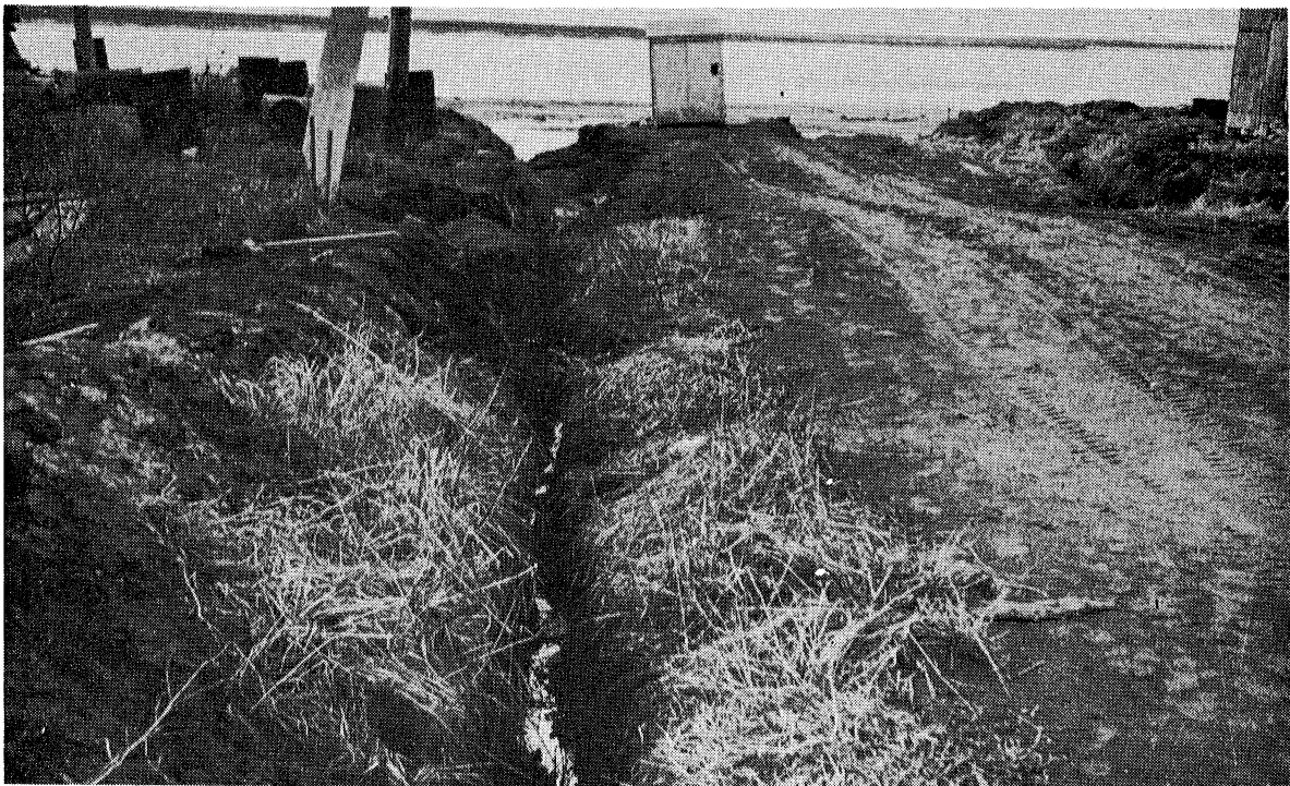
Narrow ditches are very difficult to maintain and are not recommended for areas where it is impossible to keep the ground frozen.
