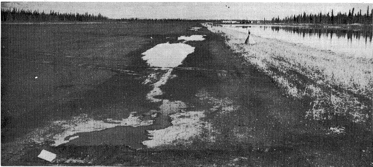
Plate No.28 - Drainage Inlets at McGrath Airfield
