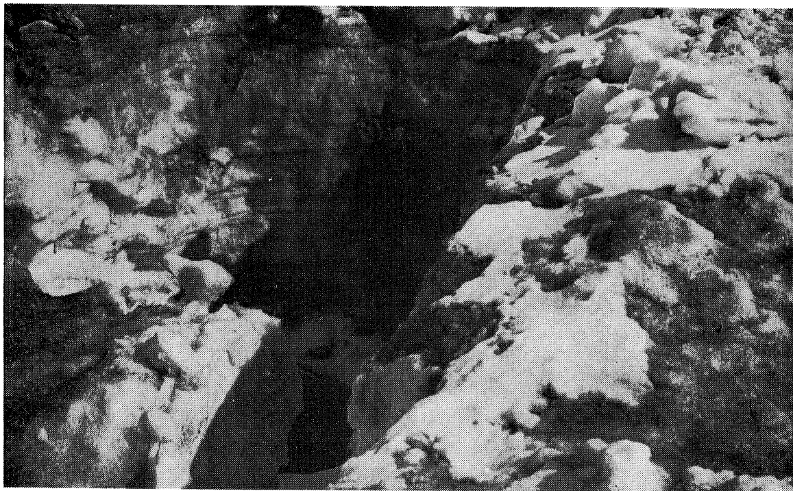
Considerable work was required to remove the ice and snow that impeded drainage into this inlet.
