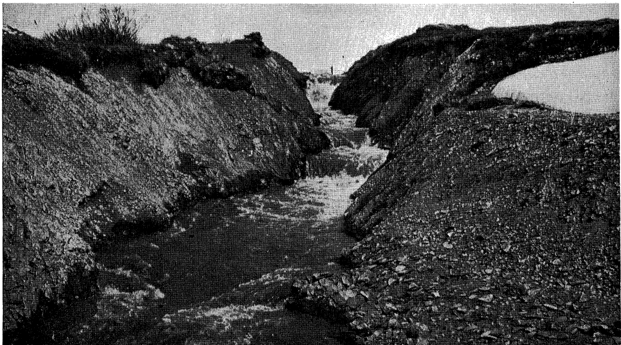
Two-thirds of the channel flow is diverted in order to carry away large volumes of floating ice.
