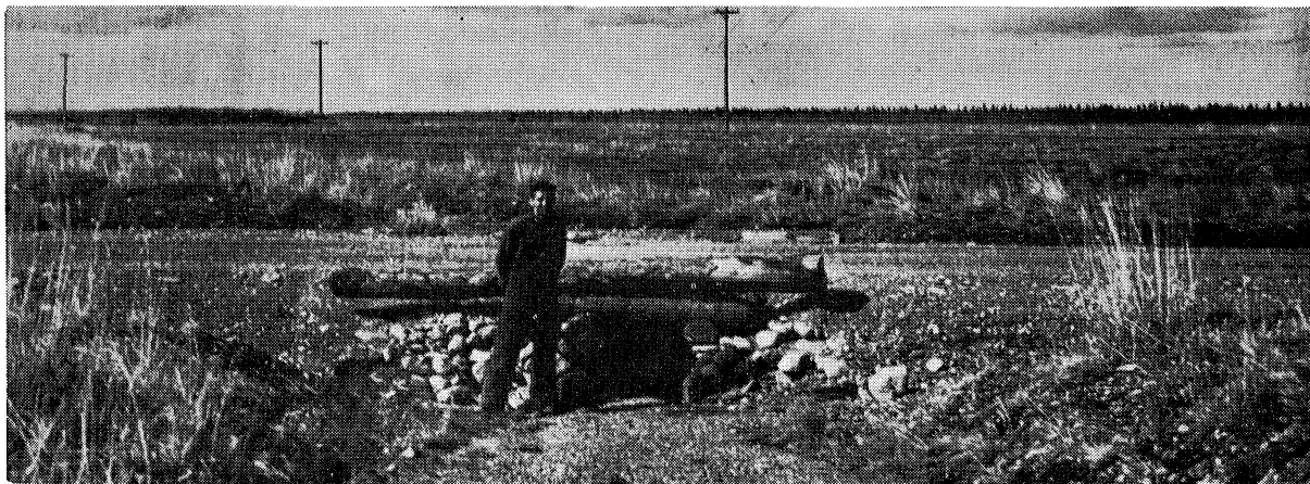
Plate No.16 - Drainage Facilities at Farewell Airfield
