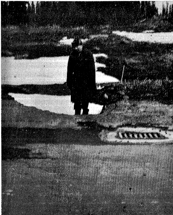
Drainage outfall structures are equipped with steam pipes to facilitate thawing.
