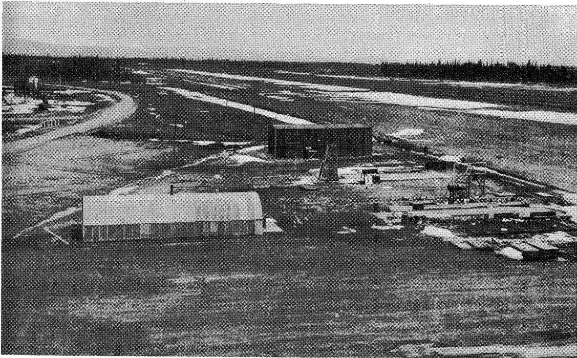
Looking northeast from the roof of the hangar.
