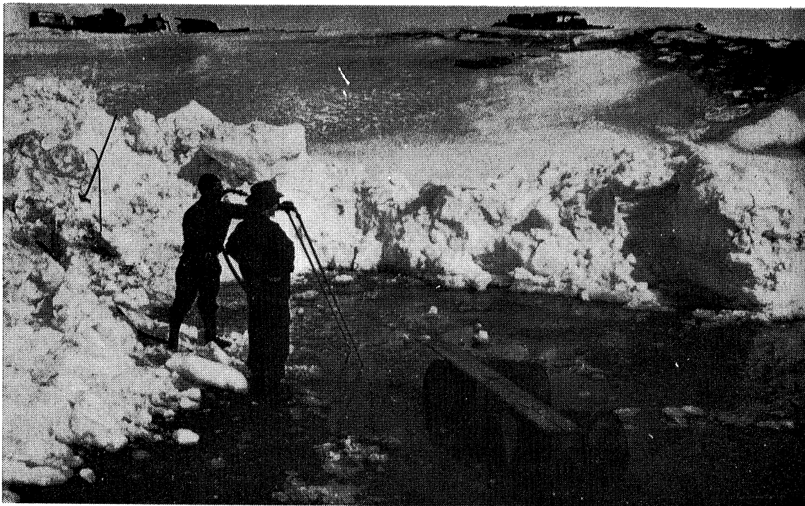
A steam-thawing operation is in progress to free a drainage inlet structure of ice.
