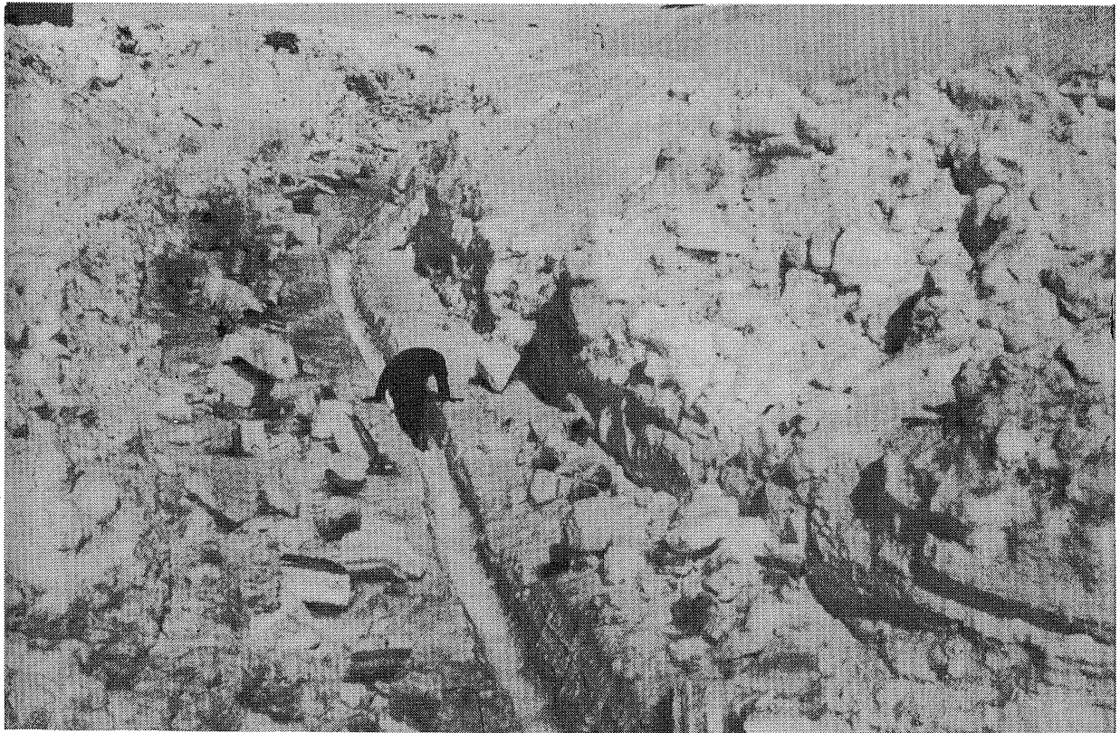
Plate No. 36 - Drainage Channels at Nome Airfield
