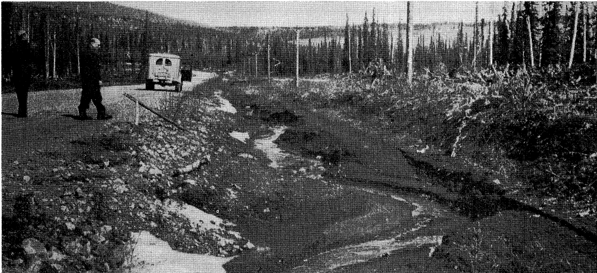
Erosion of highway ditches was quite severe in the section near Northway.
