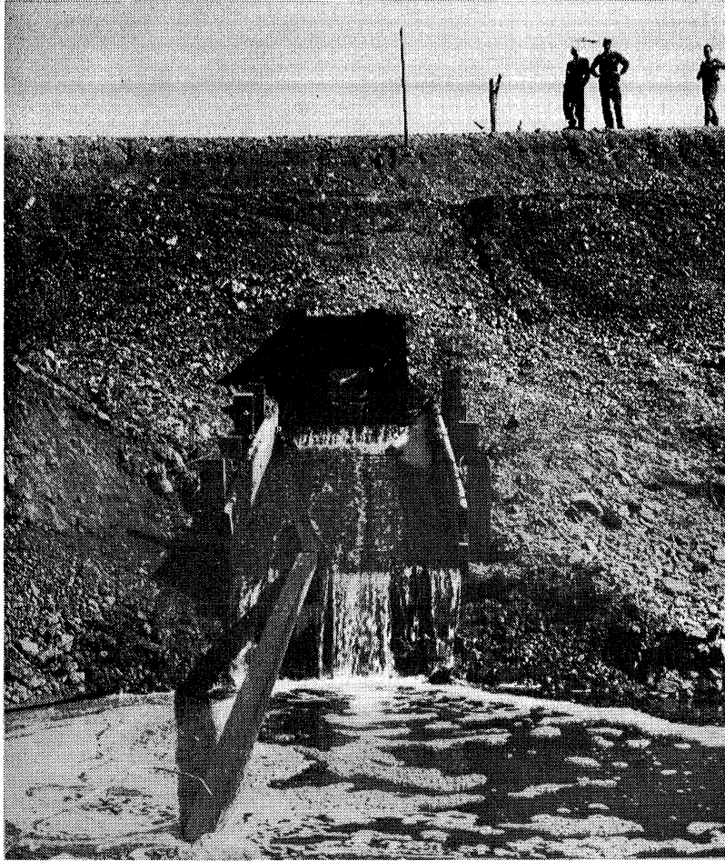
Timber box culvert near Northway.
