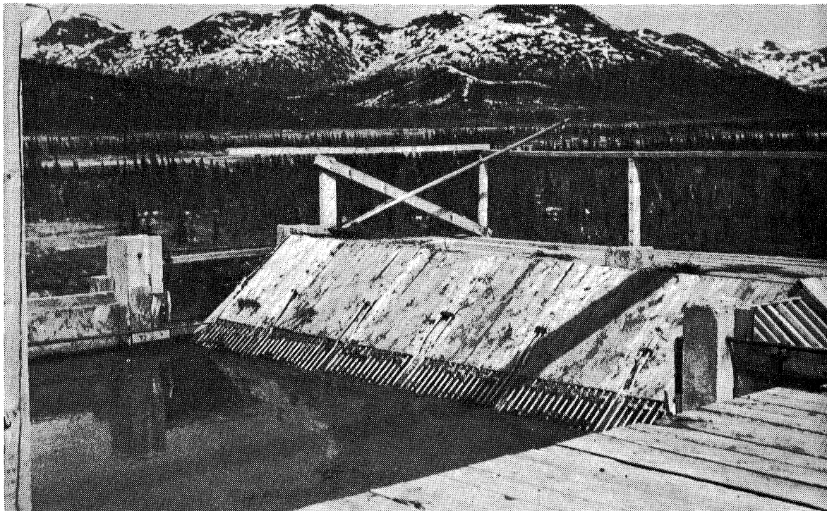
This heating element melts ice that would otherwise clog the inlet grating.
