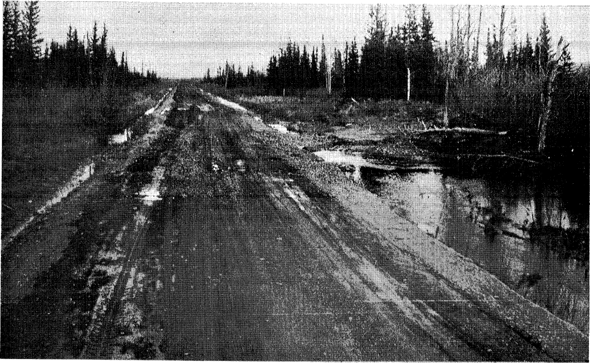
A 10-hour duration rain of May 23, 1948 resulted in considerable damage to roads.
