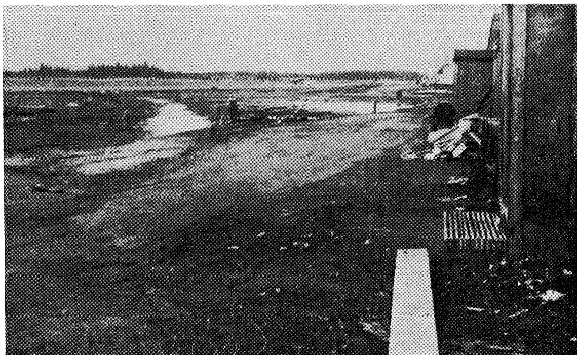
Wide, shallow drainage ditches in which heavy snow-moving equipment can operate are preferred in this area from a maintenance standpoint.
