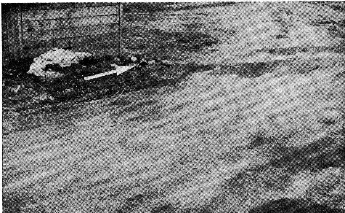
The 4-in. wooden pipe shown in the upper left part of the picture is the outlet to 10,000 sq ft of surface area.
