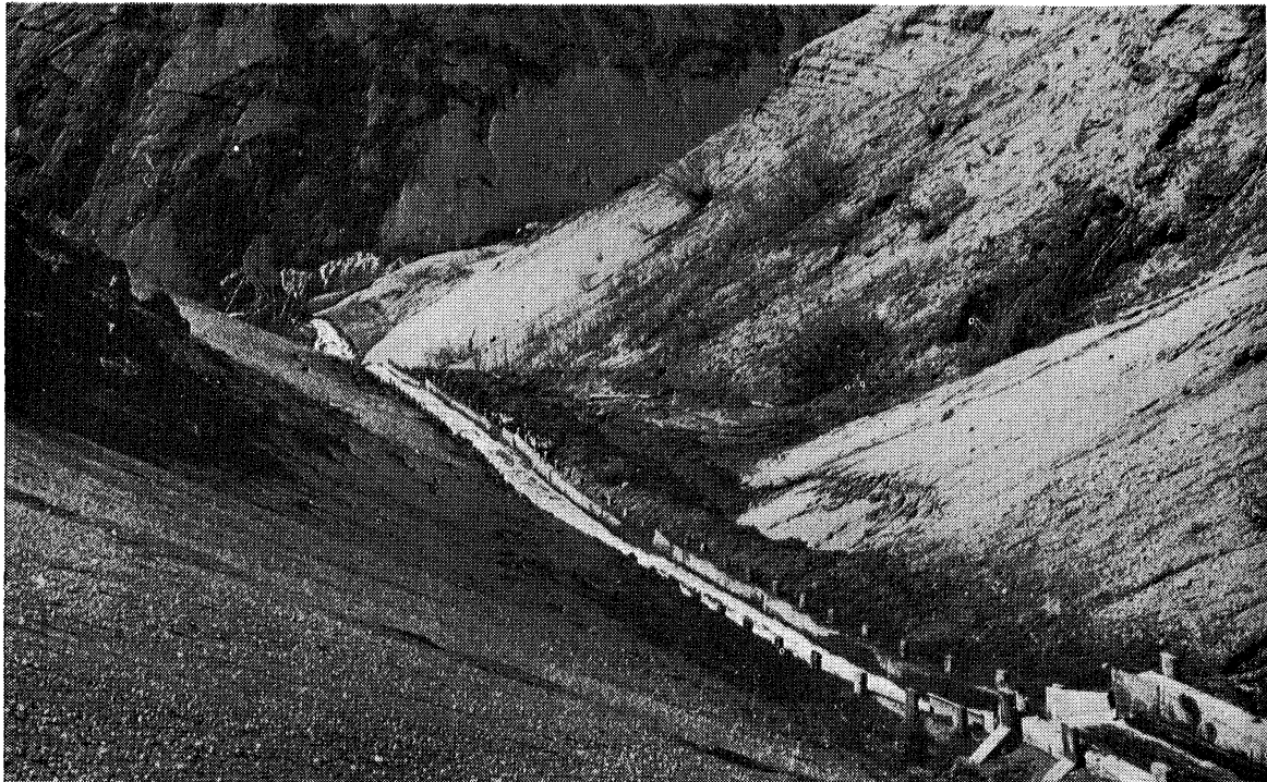
To stop erosion in this gully it was necessary to construct a long timber flume.
