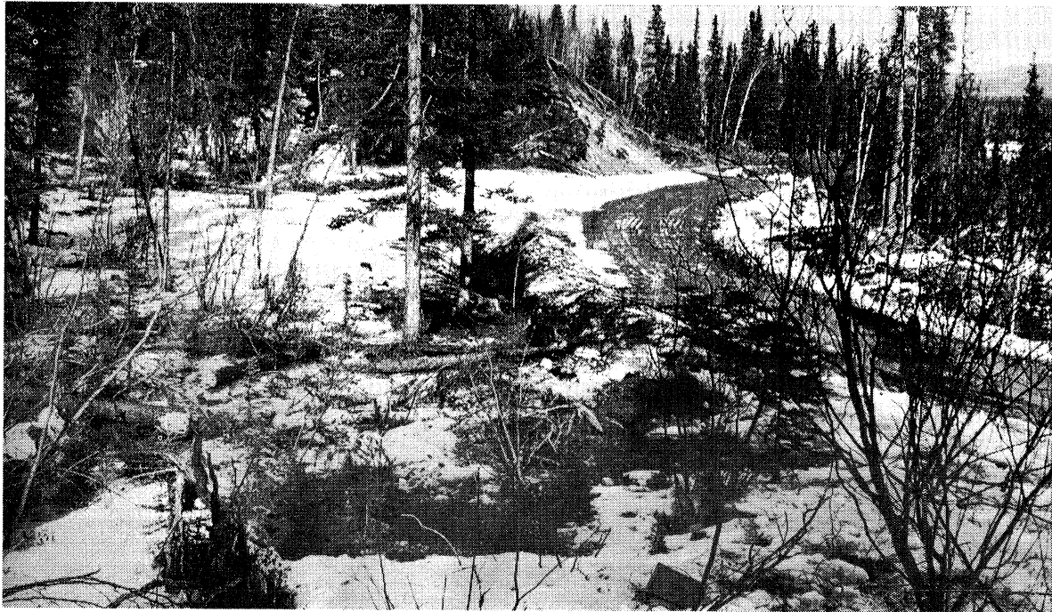
At this location it was necessary to provide drainage by blasting a channel through the ice.
