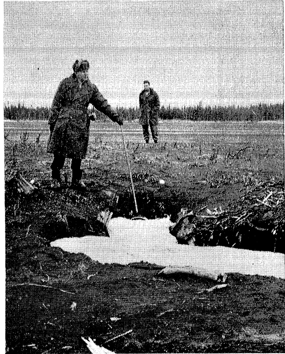
Drainage outfall structures are equipped with steam pipes to facilitate thawing.
