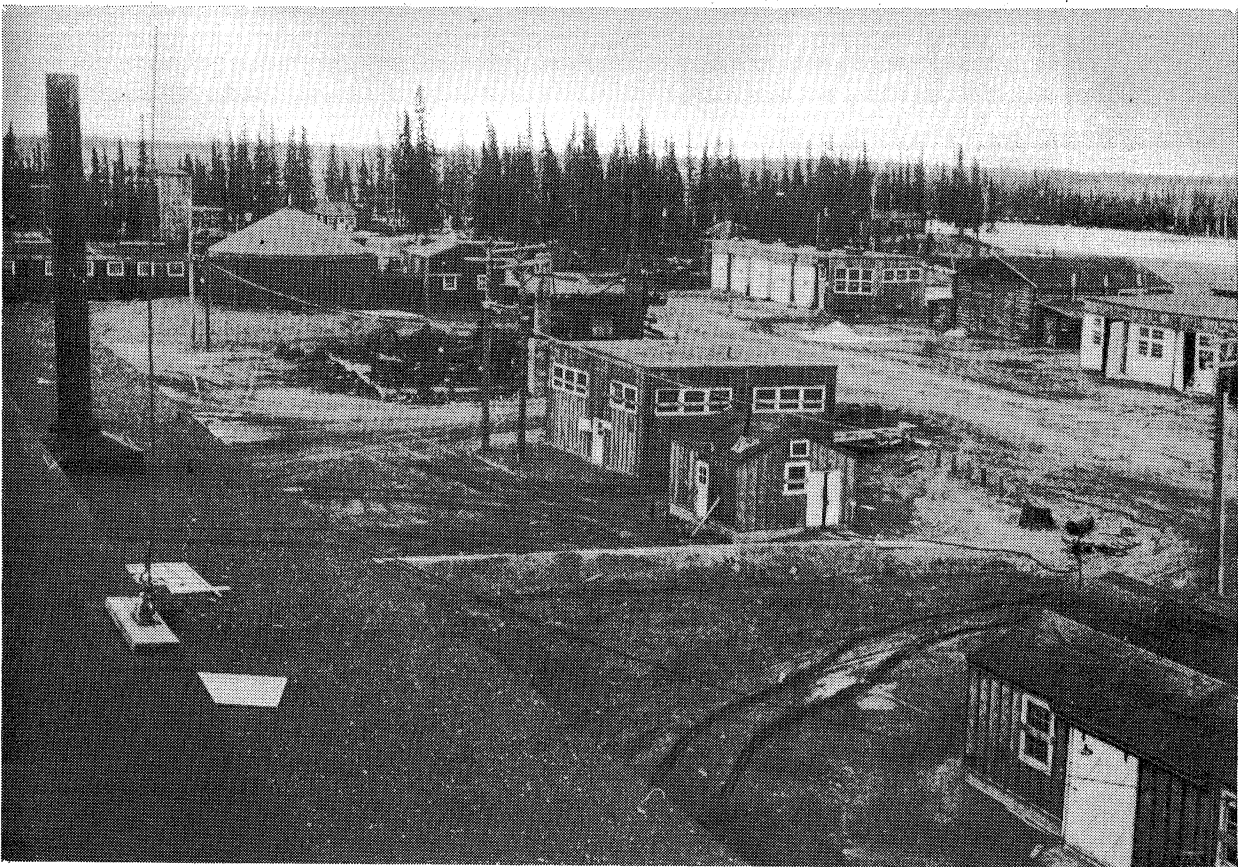
A large percentage of drainage is accomplished by proper grading. Runoff proceeds via overland flow to wide shallow ditches or to natural swales and depressions.
