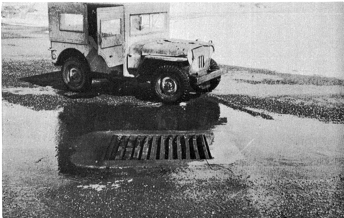
The grating for drainage inlet structures are made of light-weight railroad rails.
