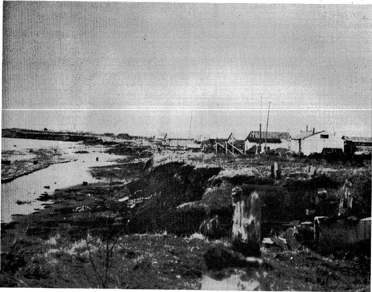
River bank erosion at Bethel is indirectly caused by thawing permafrost.
