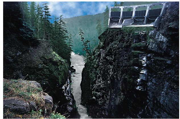
Glines Canyon before (upper) and after (simulated, below) dam removal.
