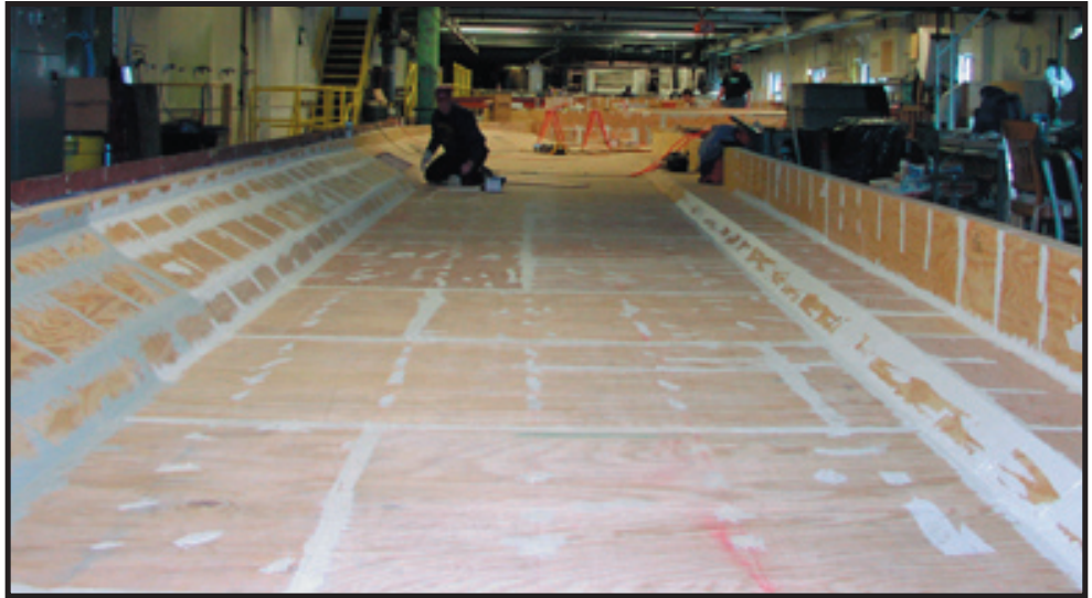
Diana Smith works on sealing the main channel of the fish bypass system model.
