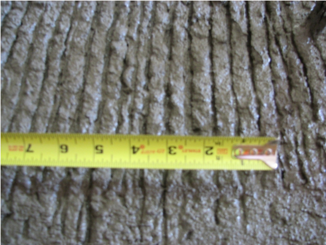
Figure 5.3.12: Intentionally roughened surface, by means of raking, of top web of precast beam used for the construction of Concept 2 laboratory bridge specimen
