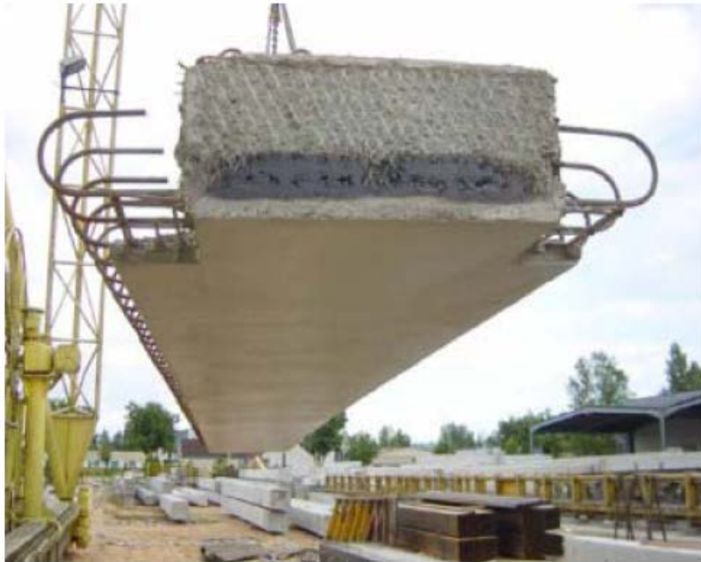
Figure 2.1.1: Photograph of precast section used in Poutre Dalle System (Hagen, 2005)
