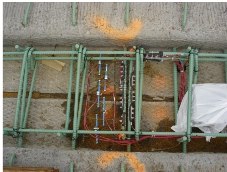
Figure 3.2.5: Lower level of concrete embedment and spot-weldable VW gages utilized in observation of reflective cracking in the Center City Bridge
