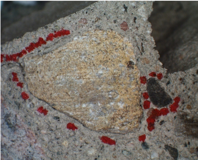
Figure E2: Identified crack marked on core specimen using red ink
