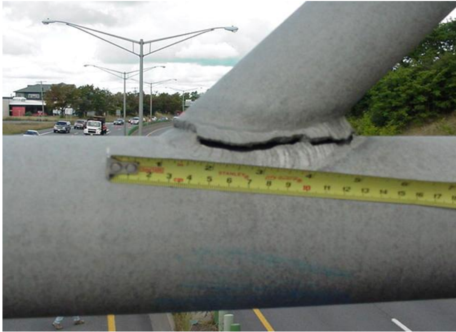
Figure 2.6 Picture of a cracked tube-to-tube welded connection.
