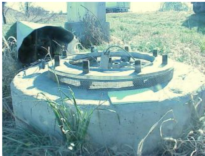
Figure 3.26 Collapsed I-29 high mast tower in Sioux City, Iowa.
