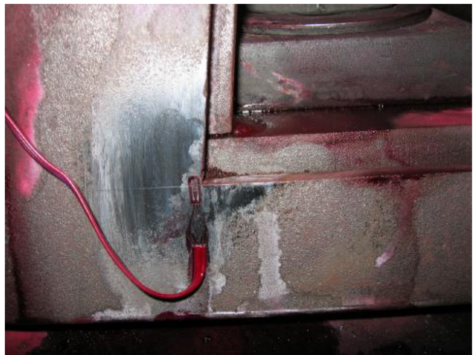
Figure 5.11 Strain gauges placed at bottom of access hole.
