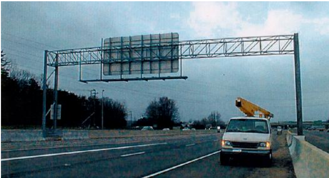
Figure 2.5 Four chord, space truss, bridged-type support using tube-to-tube connections.
