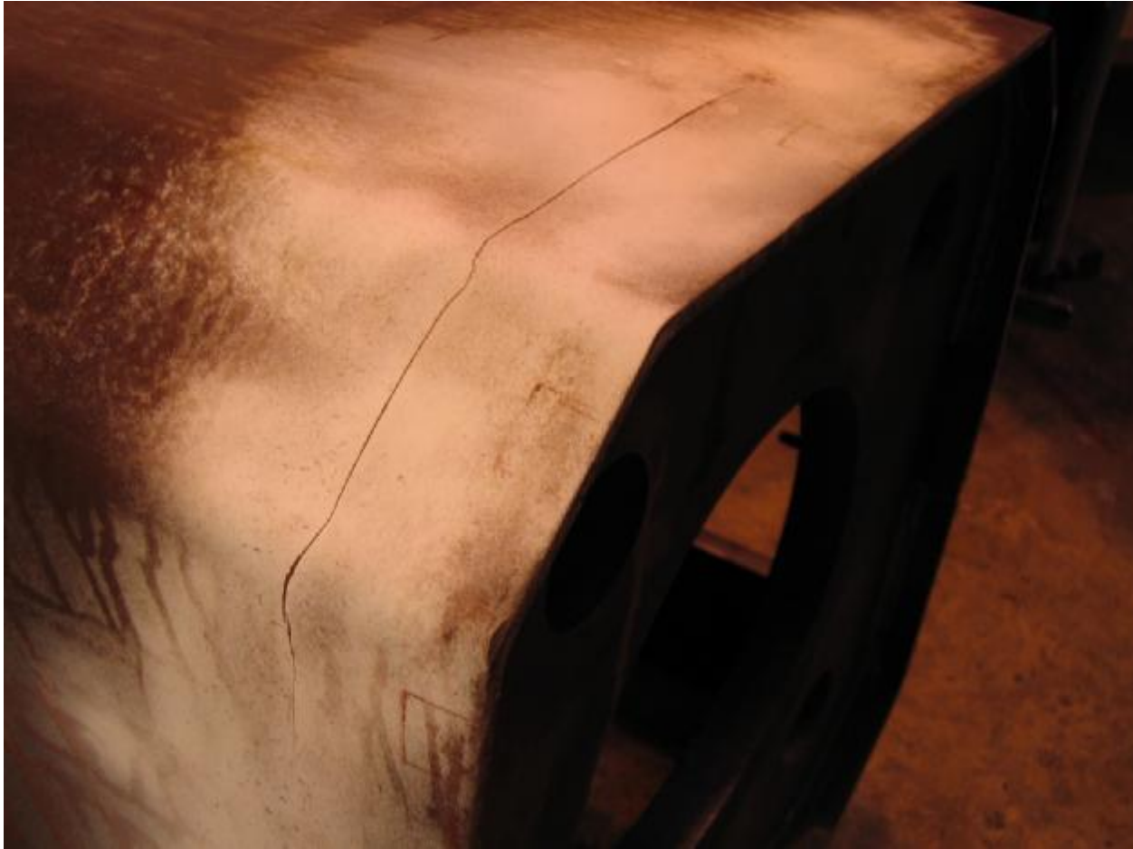
Figure 7.26 Crack in second transformer base.
