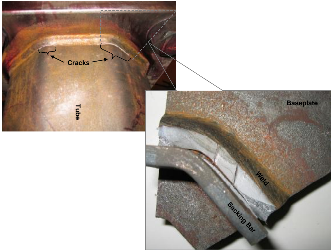
Figure 7.19 Typical cracks on Type I full-penetration weld mast arm.
