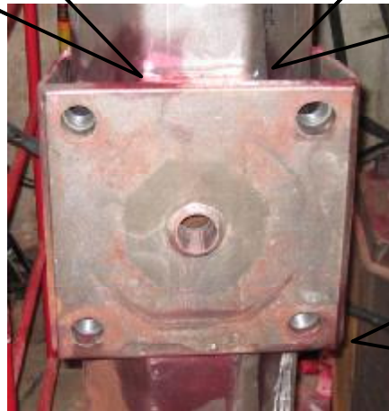
Frontal view of box connection
