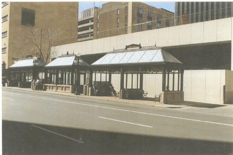
New shelters have been clustered in downtown St. Paul and begin to suggest the importance of larger scale waiting areas that describe a permanent location or station.
