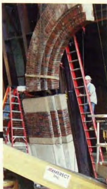
Workers piece together the sections of the Memorial Arch, creating the entrance to the Heritage Gallery.
