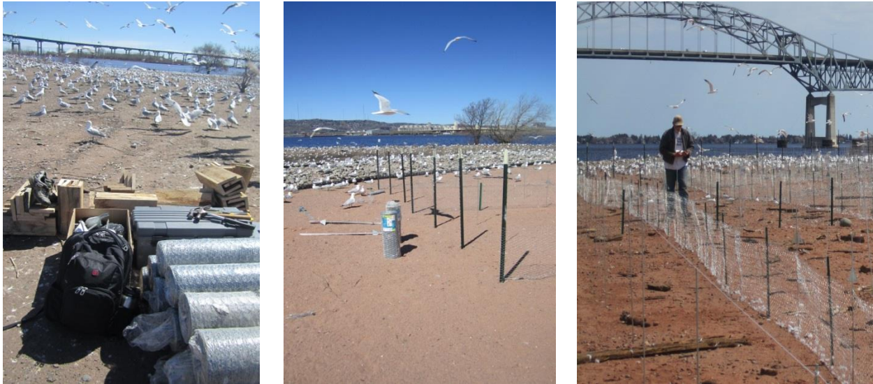
Construction of gull enclosure on Interstate Island 02-05 May, 2016. (Photo credit: A. Bracey)
