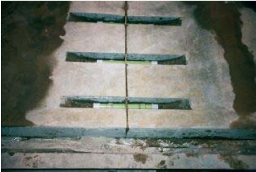
FIGURE 4-3 PHOTOGRAPH OF DOWEL BARS AND SLOTS PRIOR TO RETROFITTING
