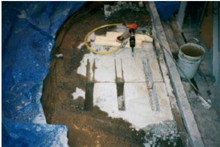
Figure 4-2 Photograph of Slot Preparation
