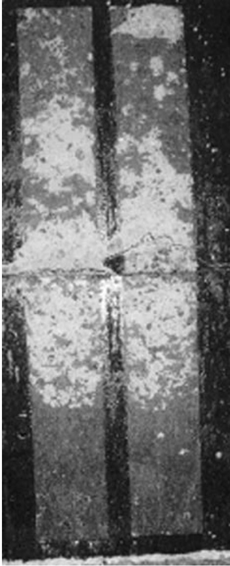
c) East Concrete
