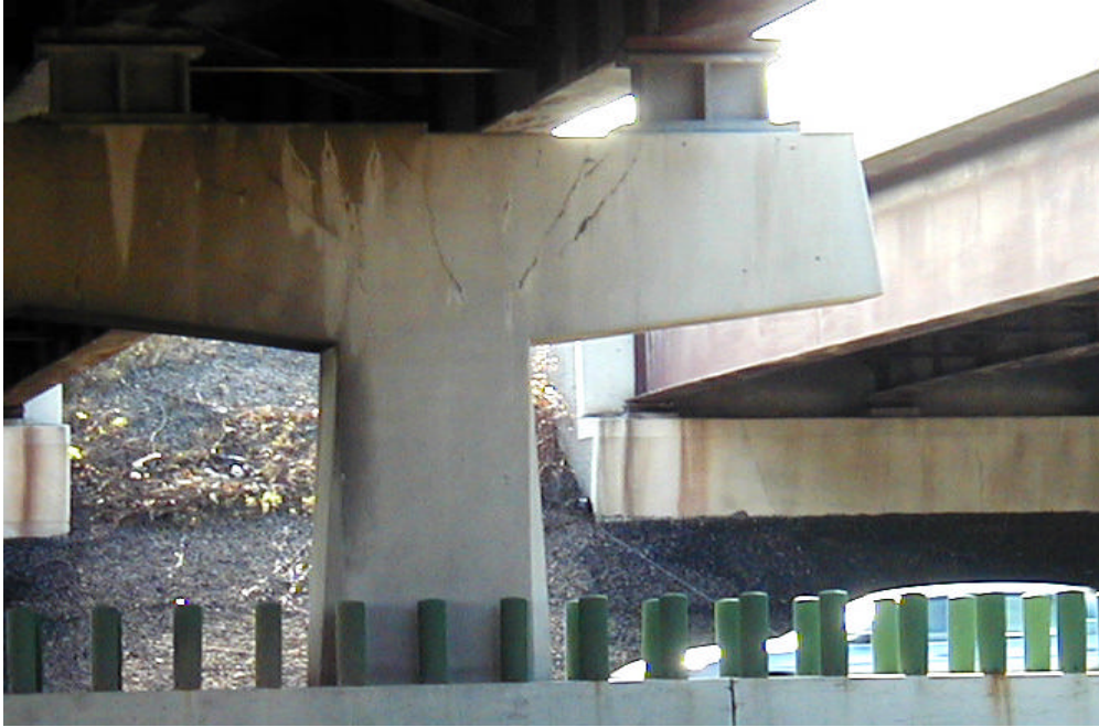
Figure 1-4 Cracked overhang of Bridge 19855.
