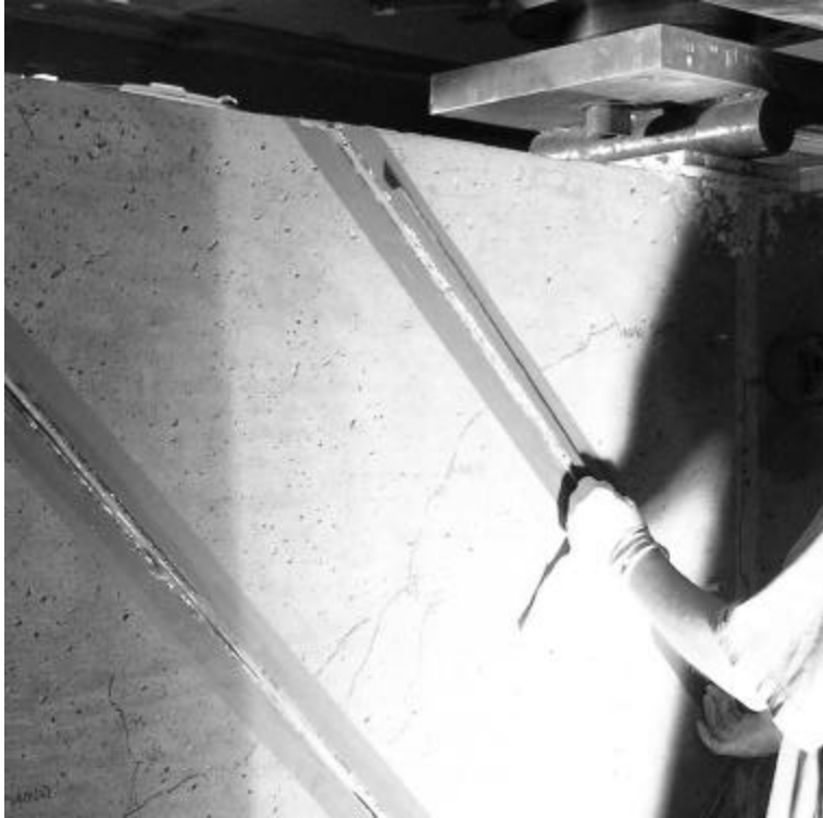
Figure G-3 Applying NSM FRP Tape into Groove
