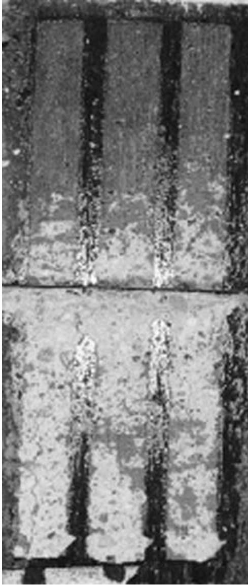
a) West Concrete
