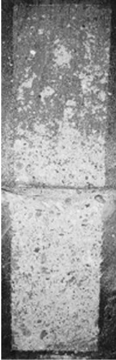
a) West Concrete
