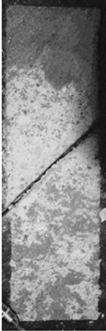
c) East Concrete
