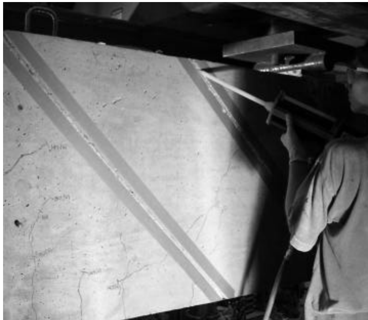
Figure G-2 Applying Epoxy
