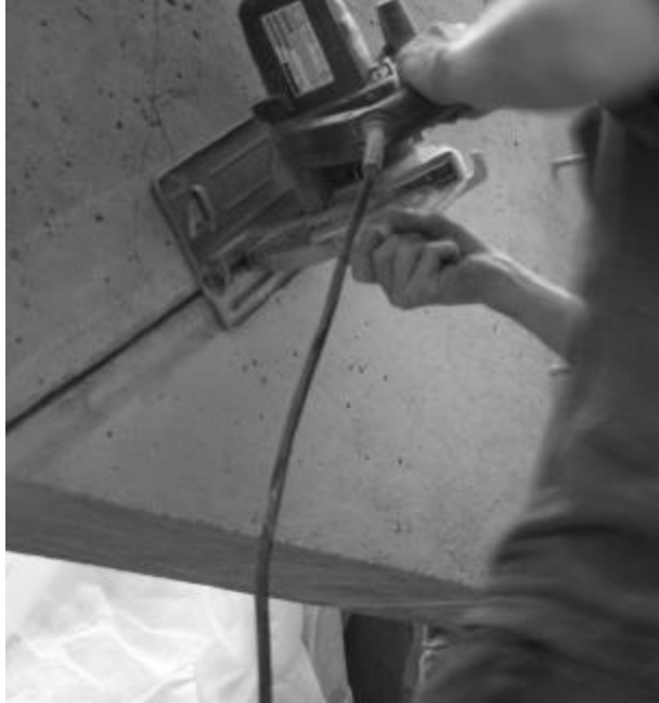
Figure G-1 Cutting a Groove for NSM FRP
