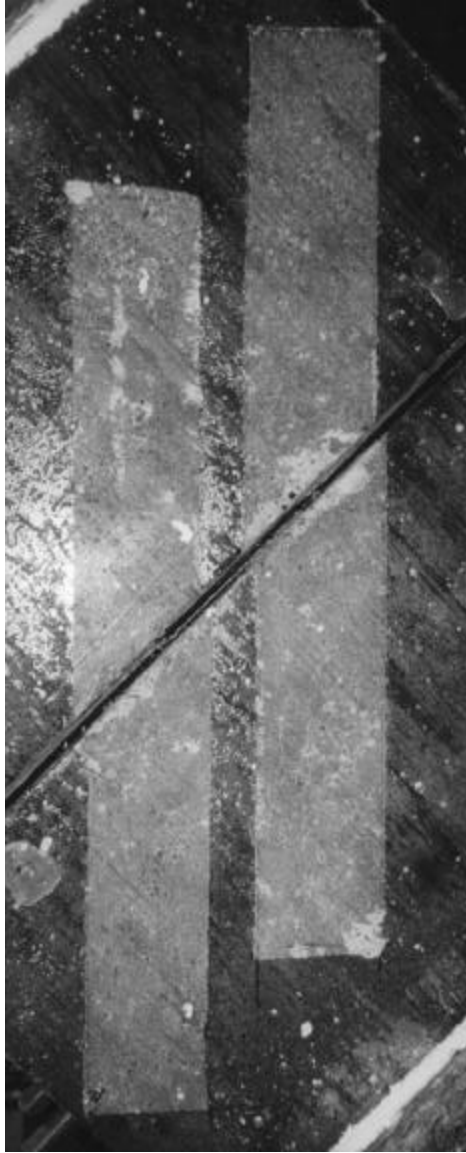
a) West Concrete
