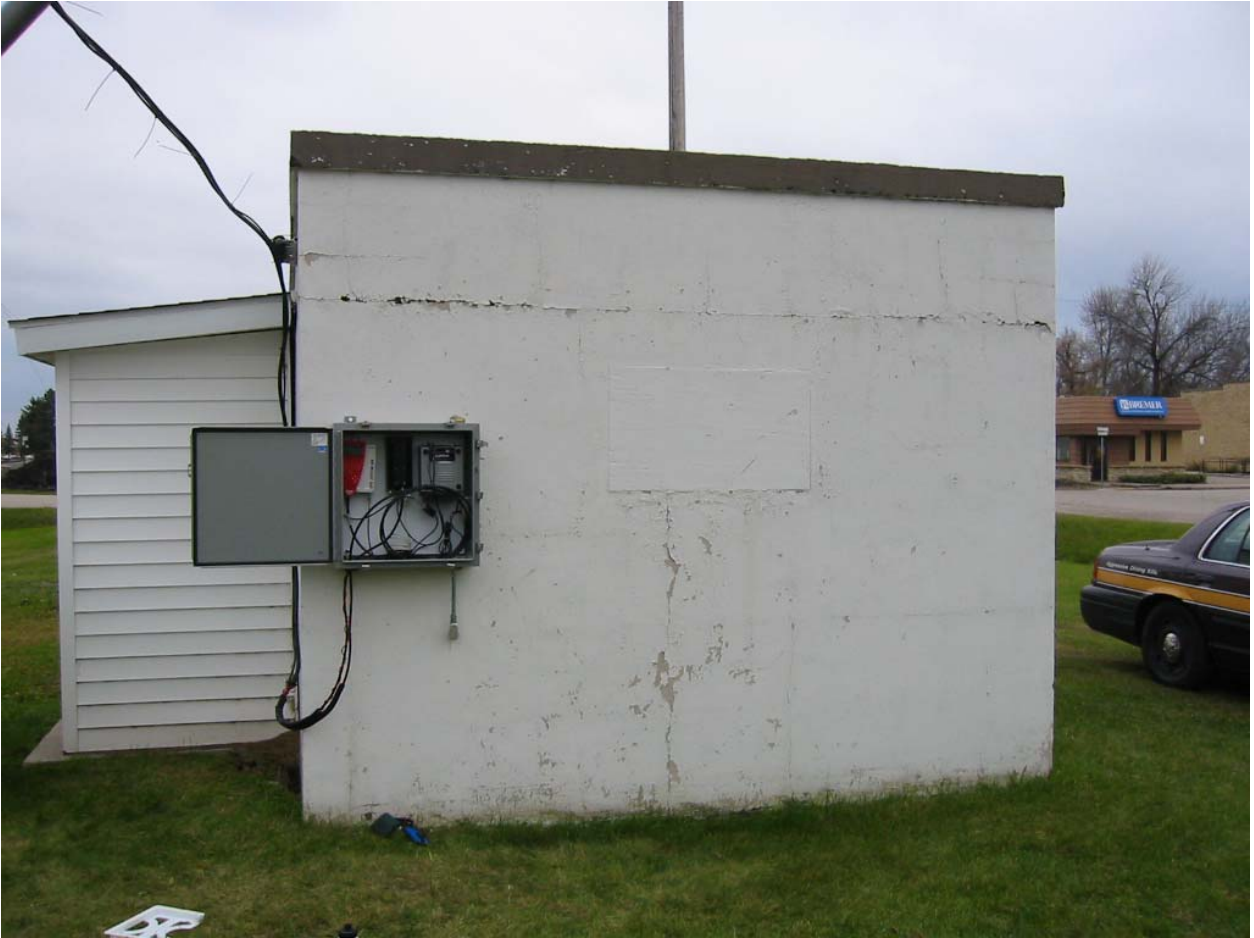
Figure 4-1. Installation of GPS base station equipment on Fisher, MN, pump house. Power to the system is provided through the conduit pushed through the pump house wall. Fisher is paid a flat fee of $150 per year to cover the expense of providing power to the system.
