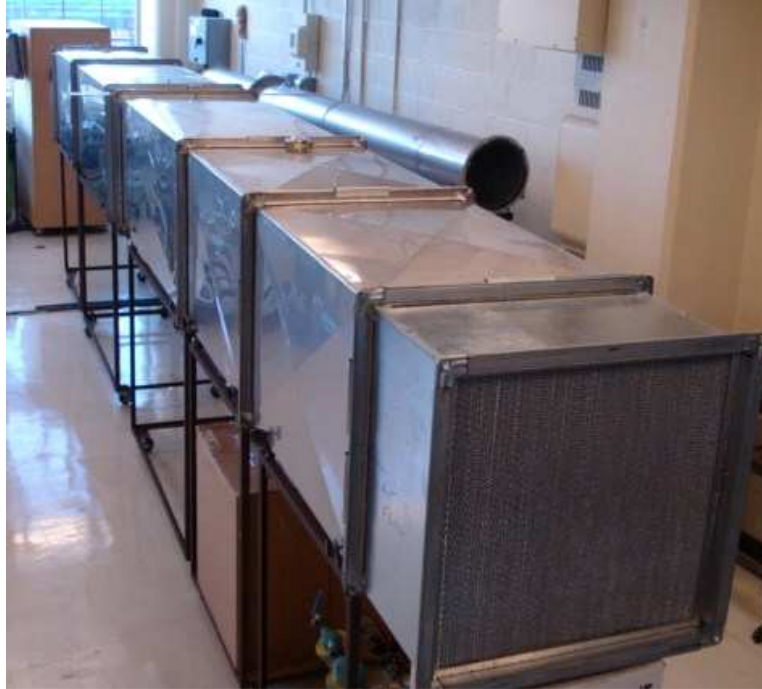
Figure 3.3.5: Picture of air handling unit without 180° bend.
