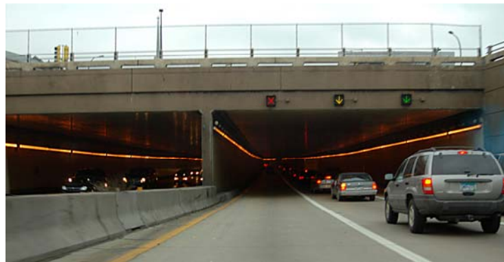
Figure 2. 1 Lowry Hill tunnel Lane Signs. Minneapolis, MN.
