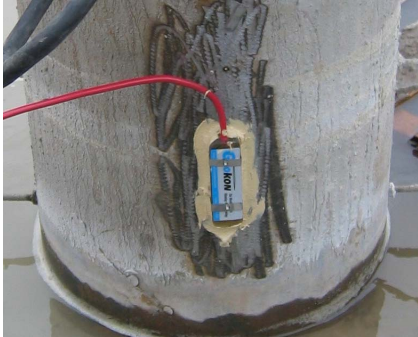
Figure 3.11. Spot-weldable vibrating wire strain gage installation on pile wall.
