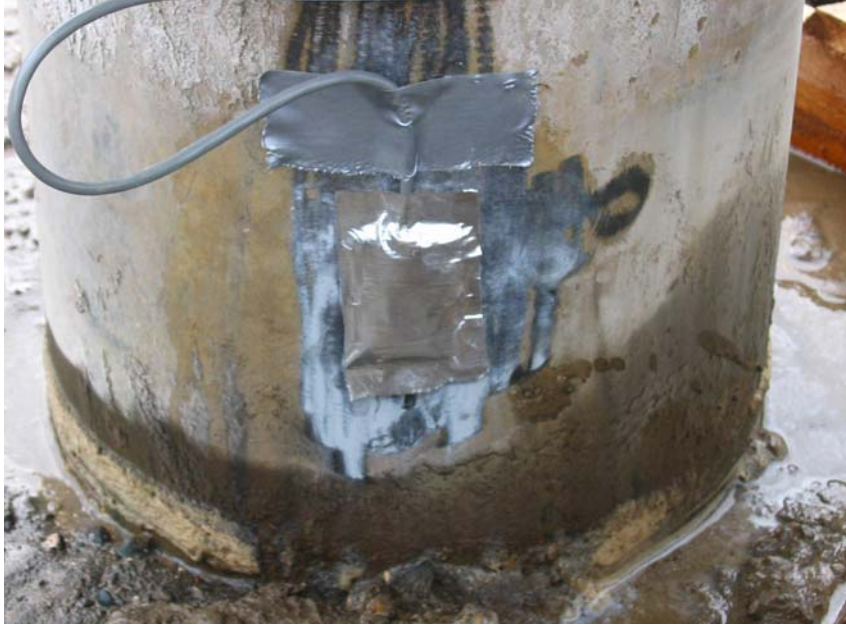
Figure 3.9. Foil gage with waterproofing on pile wall.
