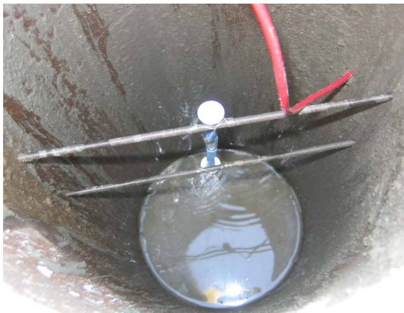
Figure 3.7. Photograph of embedment strain gage prior to attaching the coil assembly and filling the remainder of the pile with concrete.
