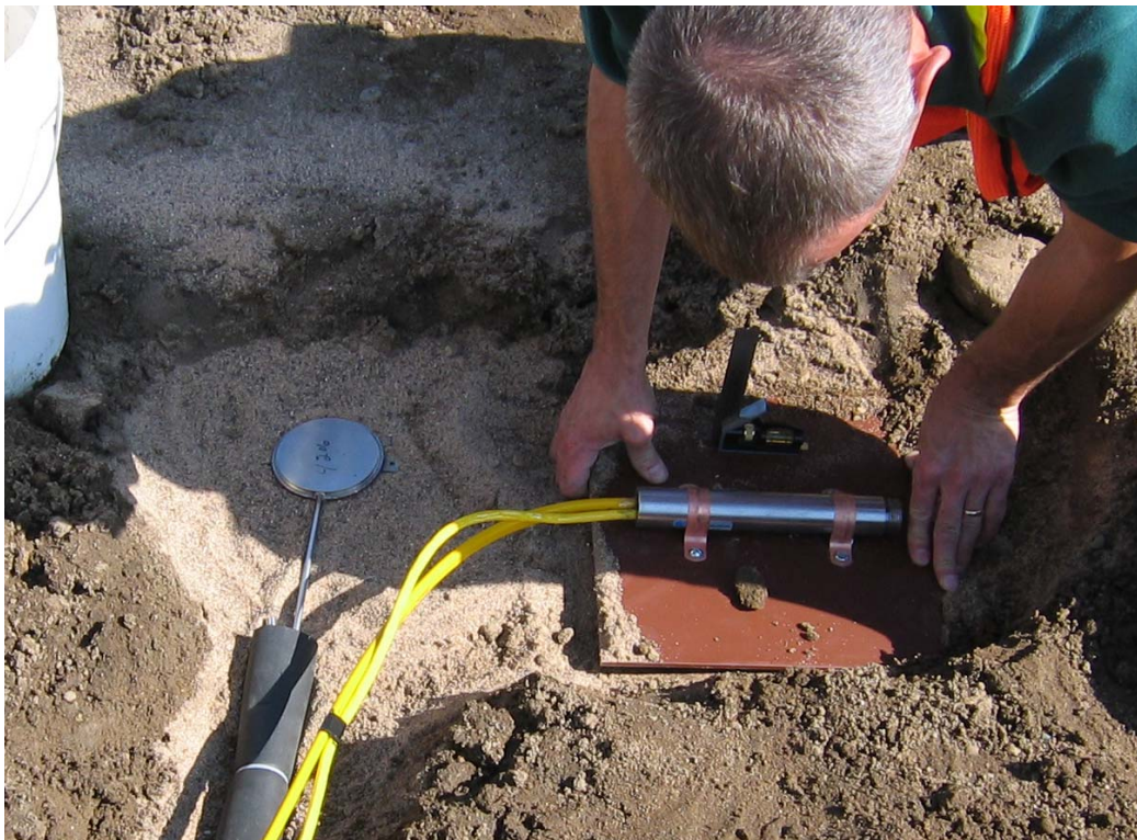
Figure 3.15. Installation of EPC (left) and settlement system (right) at the base of the LTP.
