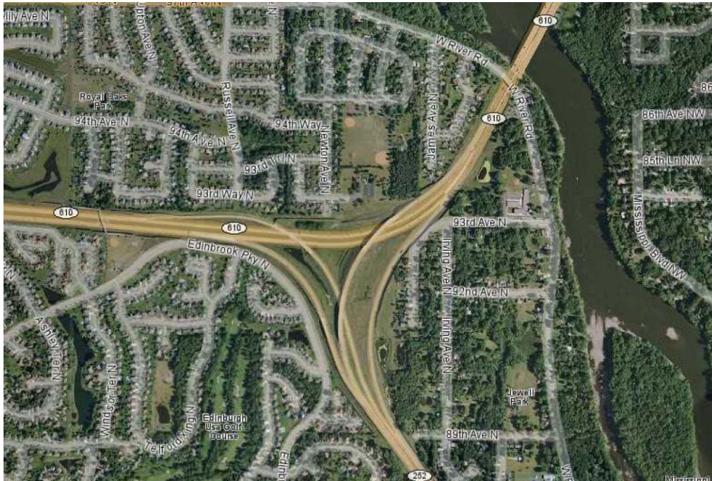
Figure 14. Aerial view of the ramps leading from both eastbound and westbound highway 610 onto highway 252 in Brooklyn Center, MN. Note that both ramps gain elevation prior to the merge point, and then drop in elevation to highway 252 grade level. The distance separating the two directions of highway 610 traffic, combined with the large geographic area creates poor visibility conditions.
