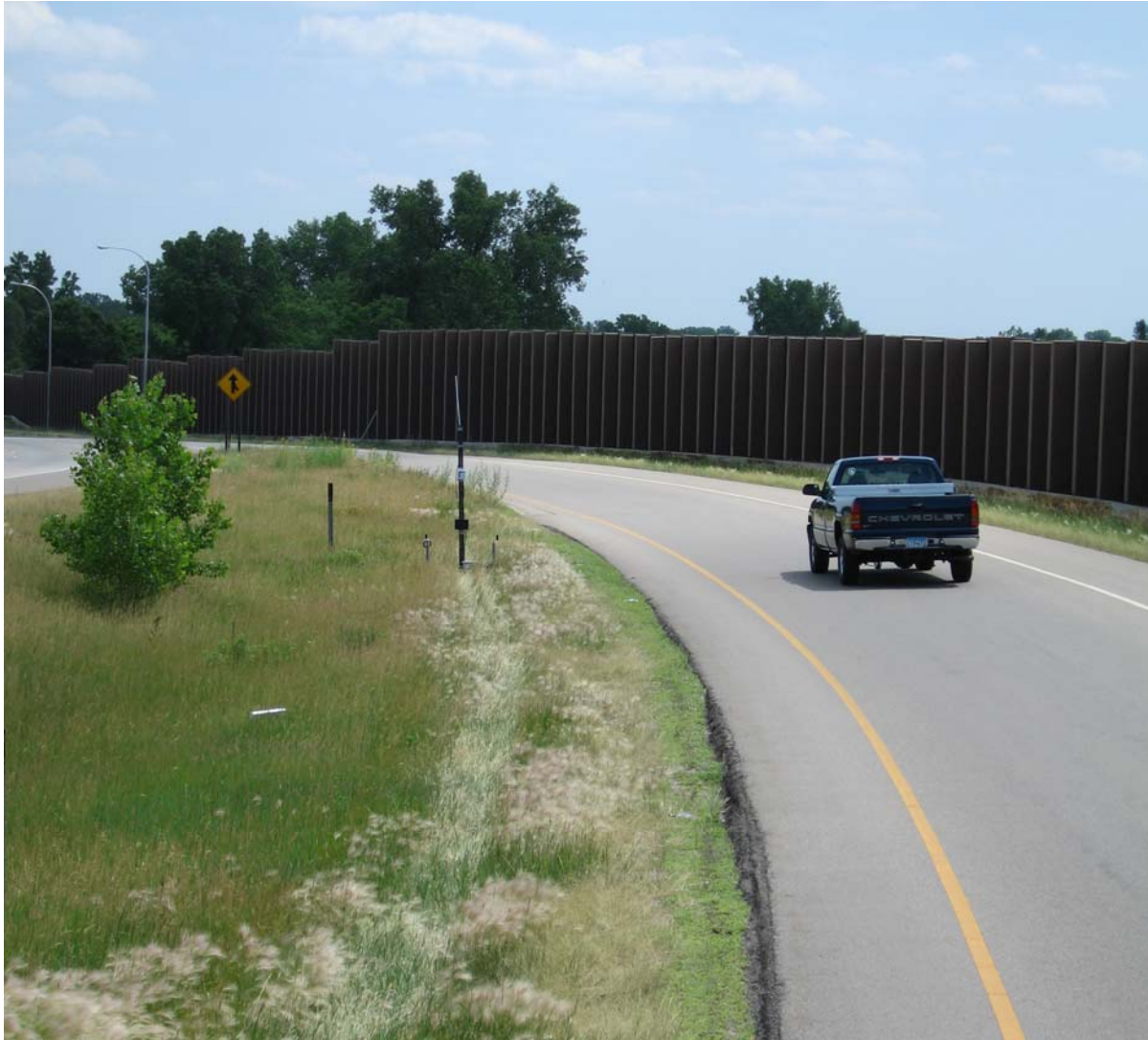
Figure 16. Picture of roadside radar sensor on entrance ramp from eastbound highway 610 to southbound highway 252. Omni-directional wireless antenna is on the top of the mast; the antenna provides direct communication to the bus. All graphic rendering is done on the bus processors.
