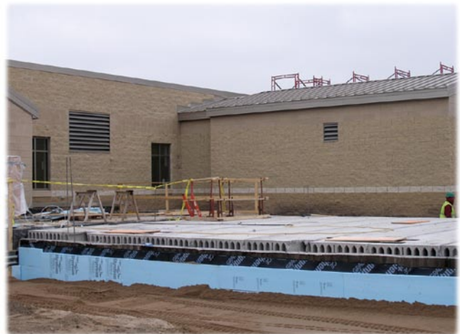
Ongoing construction site with existing BL2 facility in the back
