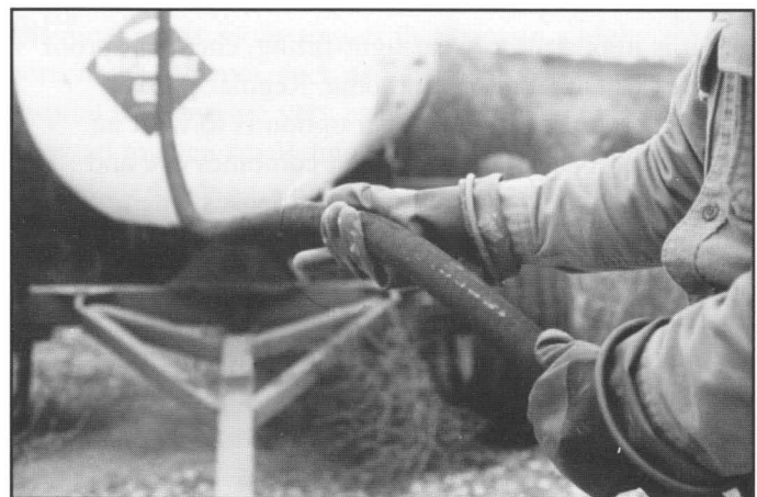
Hoses are considered the weakest link in the ammonia handling system and should be checked carefully before each use.
