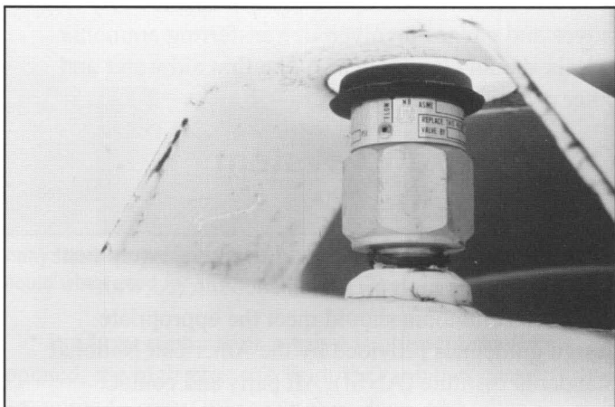
The safety relief valve is designed to relieve excess pressure from the vapor space of the tank at a predetermined start-to-discharge setting.
