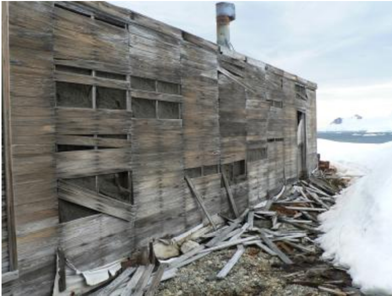
Figure 1.4. Exterior wall of former bunkhouse at East Base, with an abundance of dislodged and deteriorated wooden slats.
