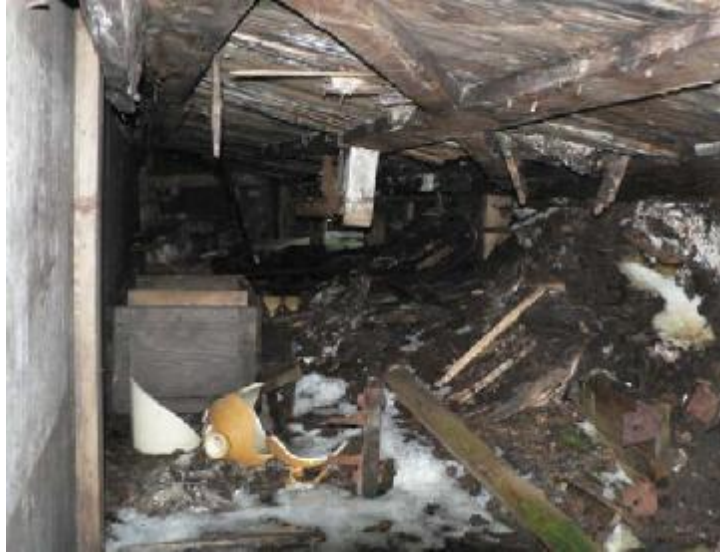
Figure 4.2. The Main Building showing collapsing floor built by British Antarctic personnel from Base E. This floor was built 4 feet above the original floor and covers historic artifacts, debris and ice.
