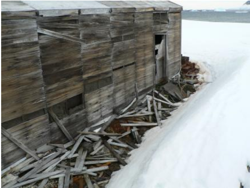
Figure 4.3. Exterior north wall of the Main Building showing the loss of many wall boards.
