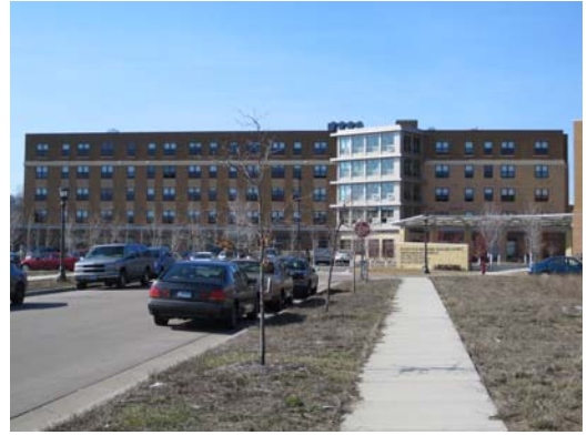
Five stories in residential neighborhood.
