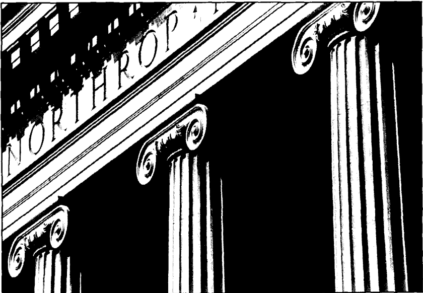
Northrop Auditorium entablature and columns
