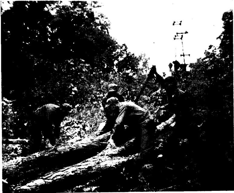
Minnesota cadets cutting timber piles for bridging.
