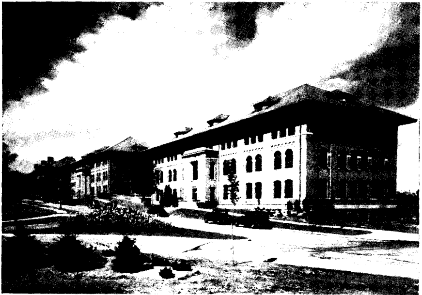
Left to right—Coffey Hall, Agricultural Engineering, Haecker Hall
