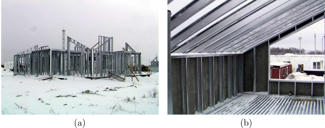
Figure 1.3. All-steel residential construction in Sorochany, Russia: (a) house under construction, and (b) close-up of the attic/roof structure ( http://profilesolutions.lindab.com )
