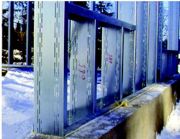
Figure 1.2. Slotted steel studs to reduce heat transfer through walls (from Reference [12])
