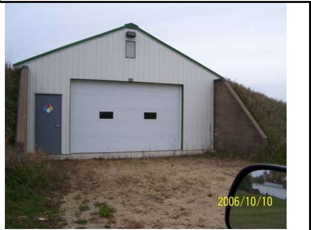
Photo 12. AOC 5. Looking East. DNT storage bunker. (1)
