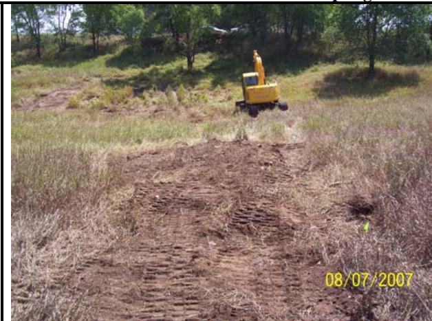
Photo 53. AOC 6. Test Pit TP5 (4)
