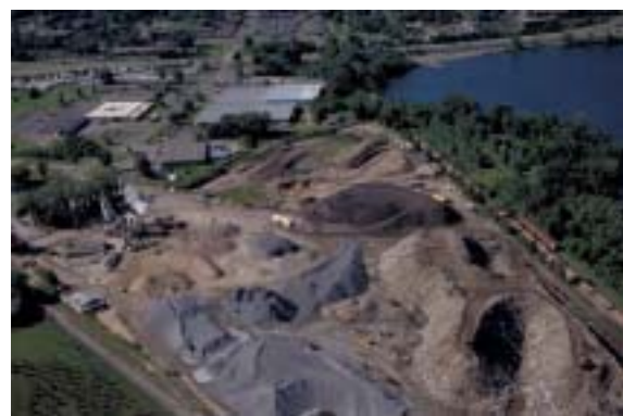
Figure 2.27. Asphalt plant in Northwest Quadrant.
