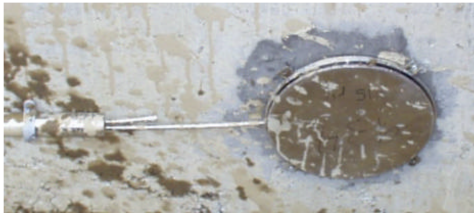
Figure 3.5. Geokon EPC attached to retaining wall.
