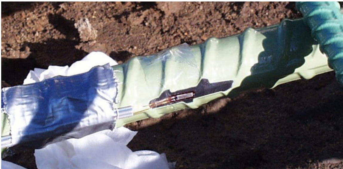
Figure 3.7. Foil strain gage attached to epoxy-coated reinforcing bar.
