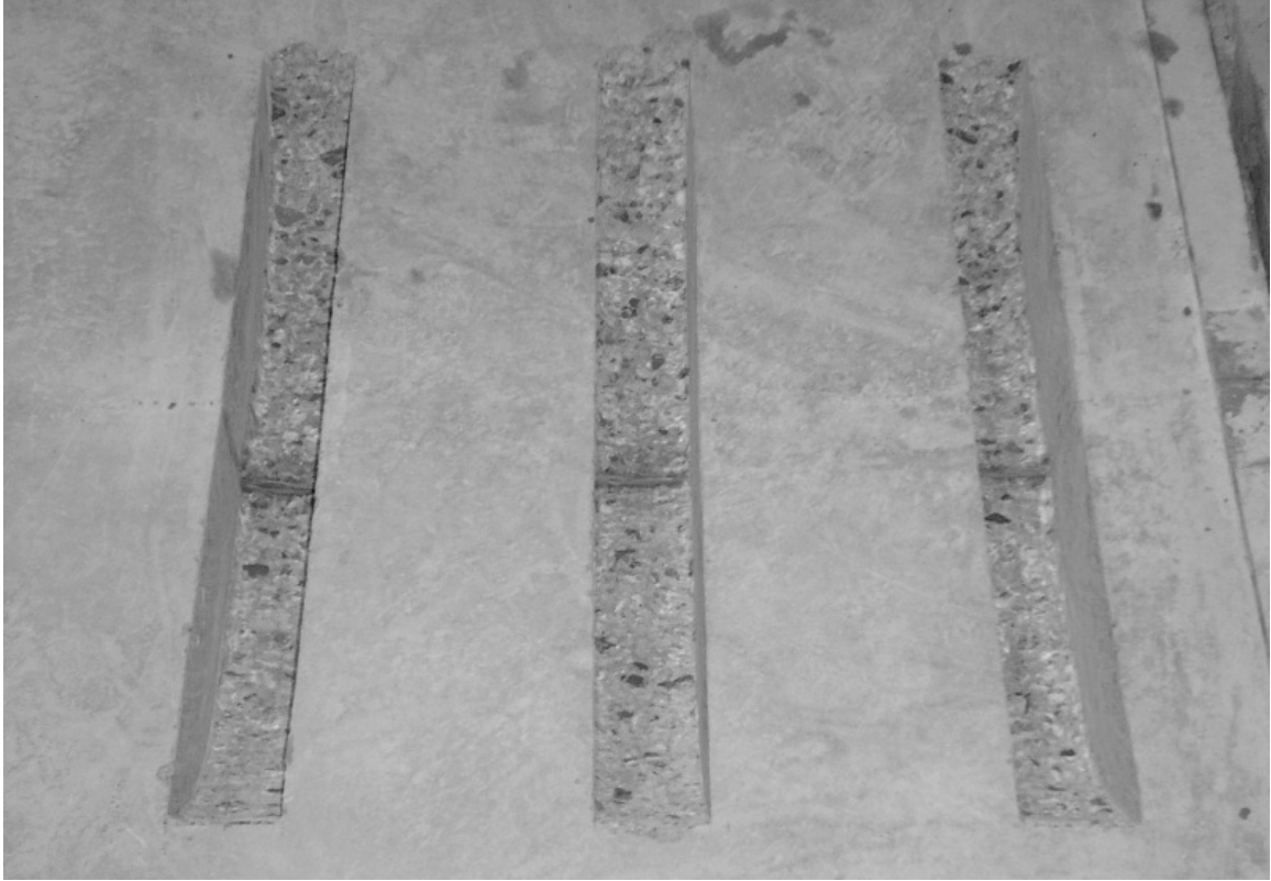
FIGURE 4-6: FINAL SLOTS AFTER REMOVAL OF DEBRIS AND CLEANING
