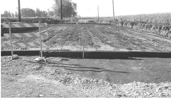
**Figure 3.5. Overlapping layers of Type V nonwoven geofabric separate granular material from wet, fine soil. 6 in. (130 mm) of Class 5 granular material protects the geofabric from the breaker run material.**
