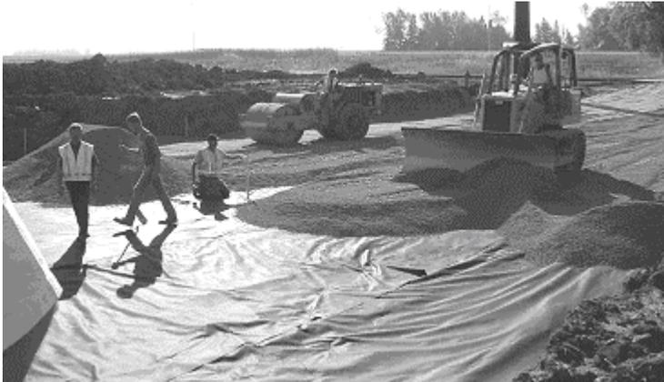
**Figure 3.6. A bulldozer spreads Class 5 material down the center while a steel wheeled roller compacts nearby.**
