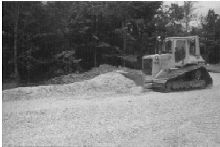
**Figure 3.9. Bulldozer spreading Lumber-Mill Sawdust**
