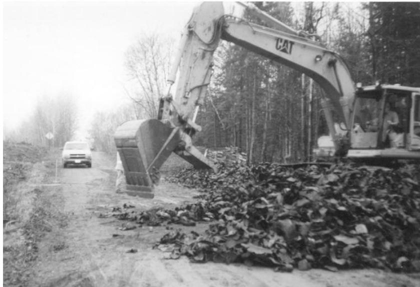
**Figure 3.13. Placing tire shreds. Loader uses a thumb-like attachment to enable grasping.**
