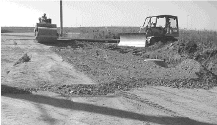
**Figure 3.7. Steel wheeled roller applies compactive effort to a 9- in. (230-mm) lift of Breaker Run Limestone.**
