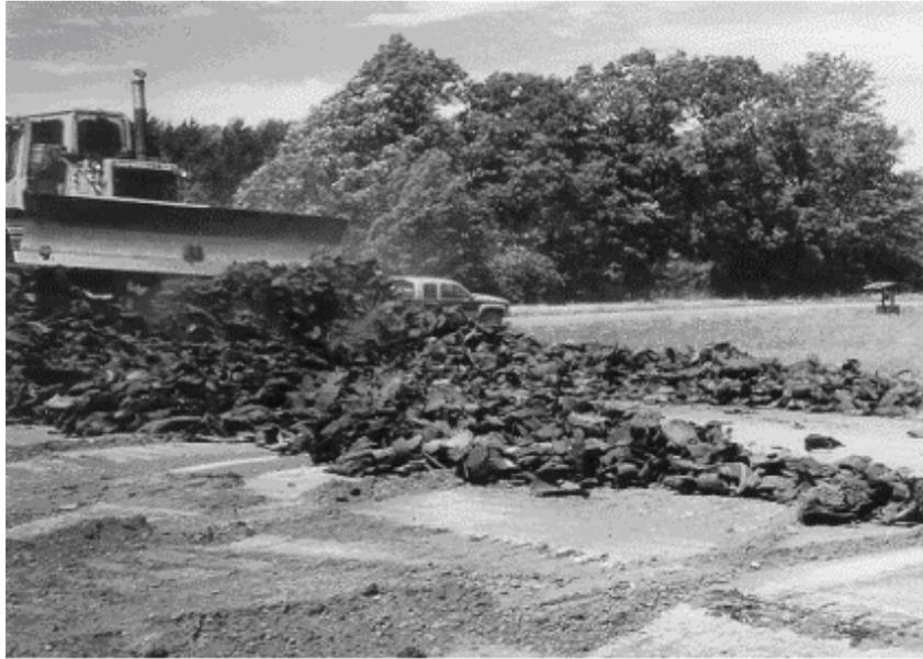
**Figure 3.14. Loader distributing and compacting tire shreds.**
