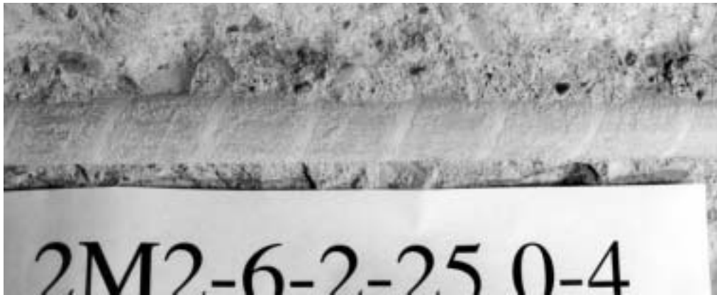
Figure 3.49 M2, Bar Impressions in Concrete
