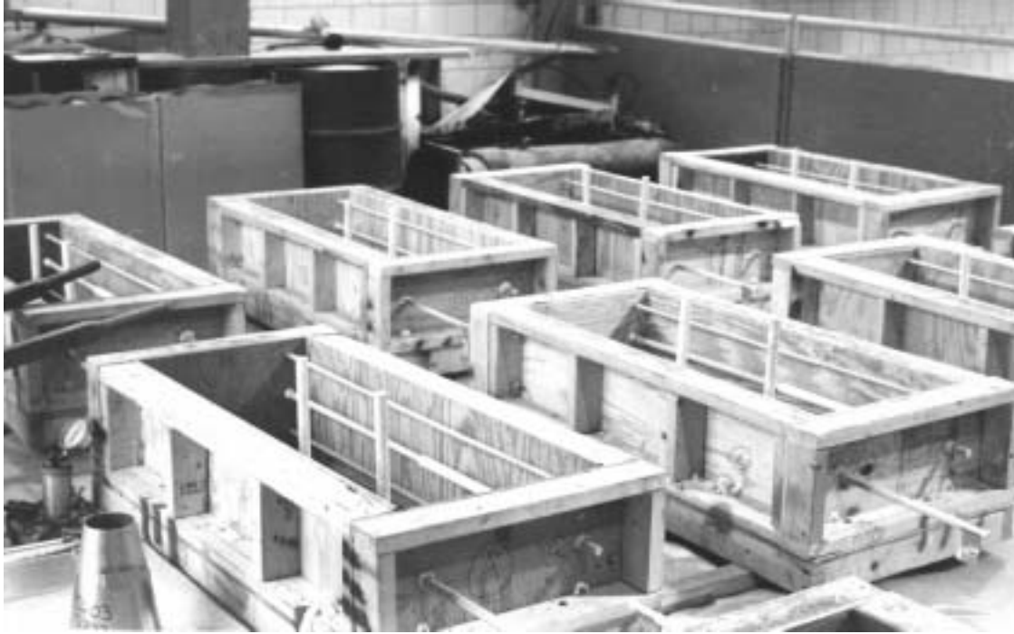
Figure 2.8 Concrete Specimen Forms
