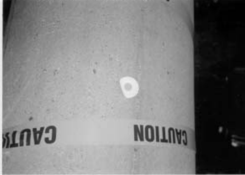
Figure 5.15: Installed moisture sleeve
