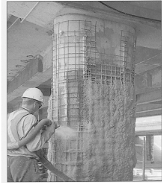
Figure 3.13: Cellulose fiber application on a column in Regina, SK, Canada
