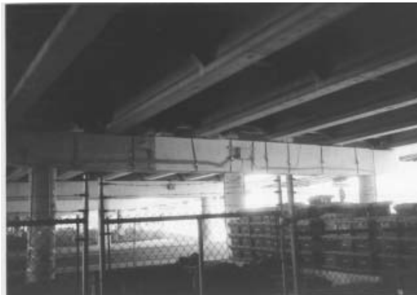
Figure 5.14: Instrumentation wiring system on Pier 34 North
