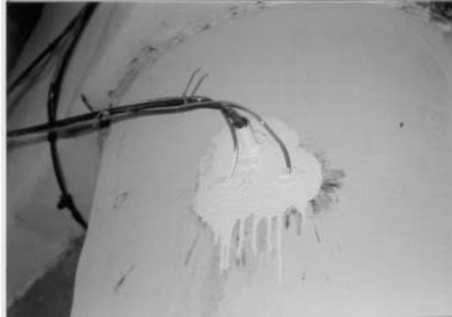
Figure 5.13: Installed and sealed corrosion monitoring instrumentation
