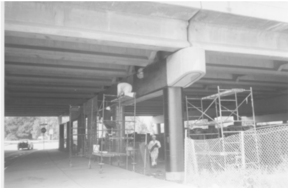
Figure 3.19: Installation of AMOCO CFRP in progress above Column 34F
