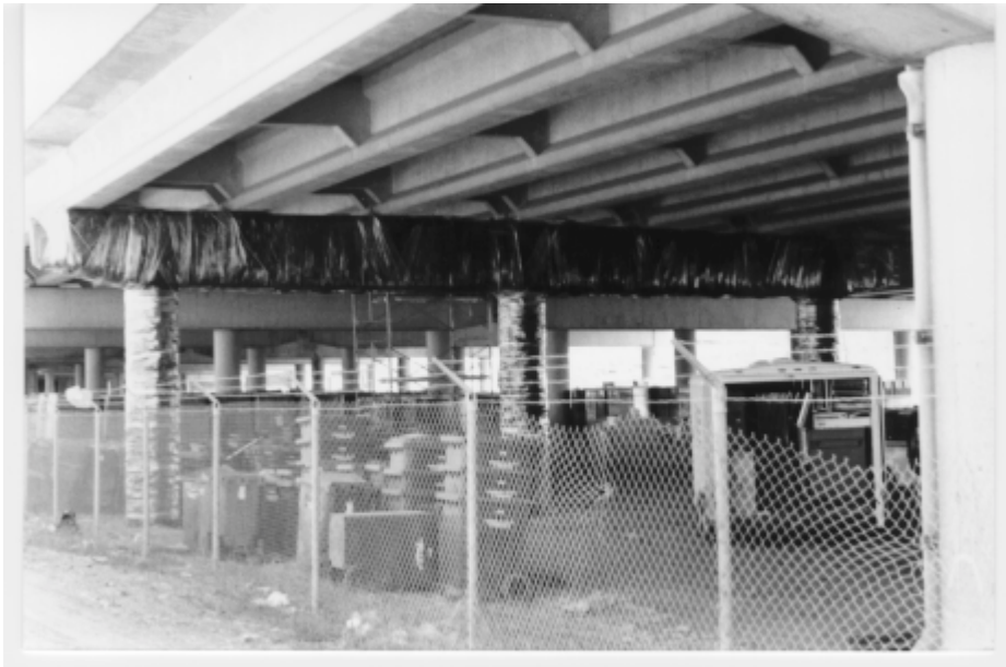
Figure 3.15: ECE system in place on Pier 37 North
