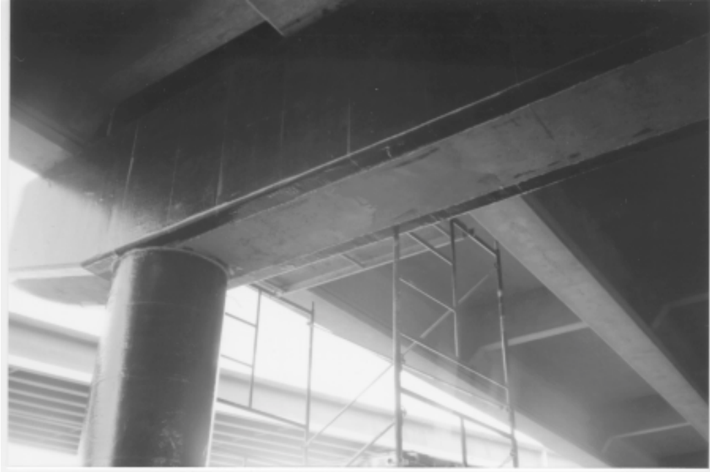
Figure 3.20: Caulk seam at top of column and drip ledge along wrap overlap
