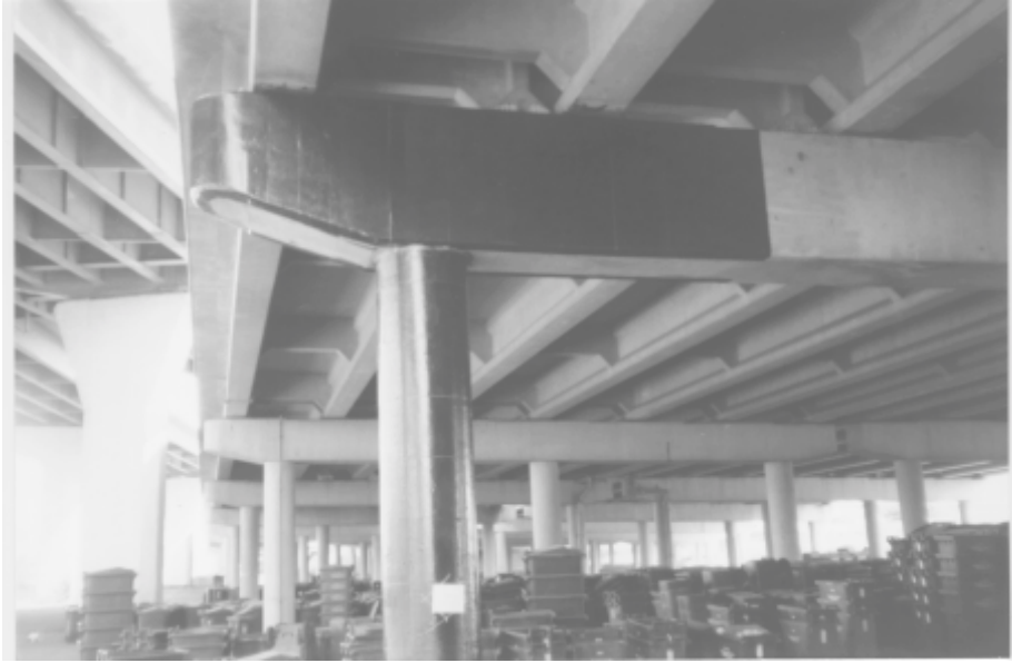
Figure 3.18: MBrace CFRP in place on Column 40A
