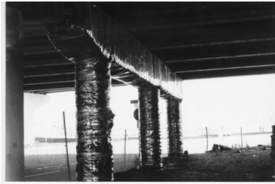
Figure 3.14: ECE system in place on Pier 34 North
