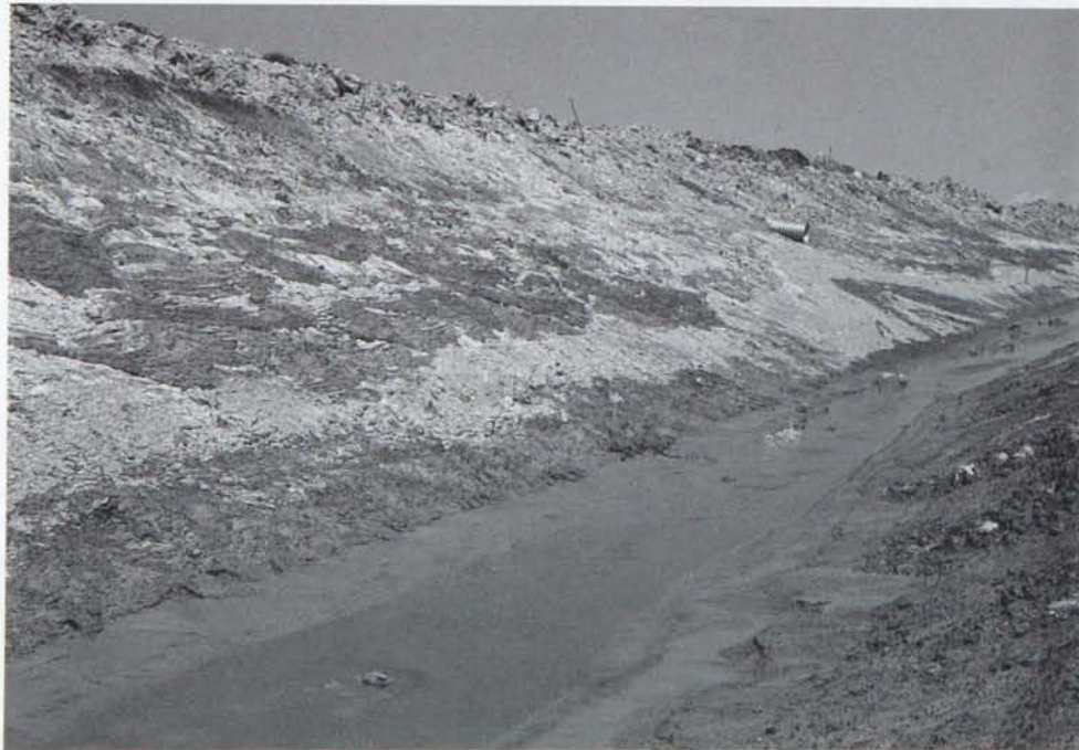
Figure 4. Exposed varves in Swift County ditch 22 (branch 6, lateral 1 of County ditch no. 22, located 8 miles north-northeast of Montevideo - T. 118 N., R. 39 W., secs. 29 and 30). Culvert for scale; the ditch is approximately 12 ft deep.
