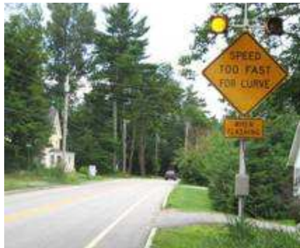
Figure 3.4 Dynamic Curve Speed Warning Sign (with a flashing beacon and radar detection)
