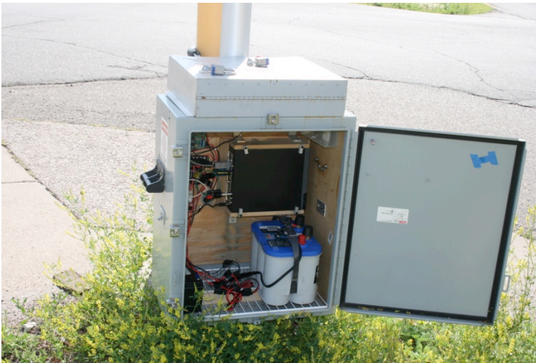
Figure 2: The cabinet with mounted components.
