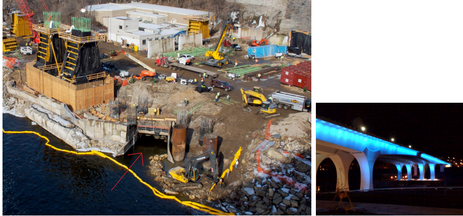
Figure 1.1: Example Modification: 35W Bridge, Minneapolis
