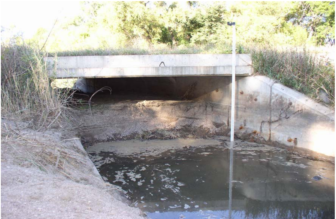
Figure 6.2. Sediment accumulation in a box culvert at U.S. Army Corp of Engineer’s bridge #23 in the Upper watershed of the South Fork Lac qui Parle River.
