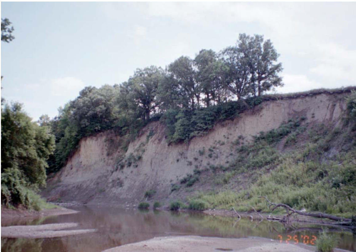
Figure 4.11. Downstream view at XS-128 illustrating the steep bluffs found along the SF LqP River in the Lower watershed. Soil material is actively eroding into the SF LqP River due to erosion at the toe-of-slope. Vegetated area in foreground is a remnant slope failure.
