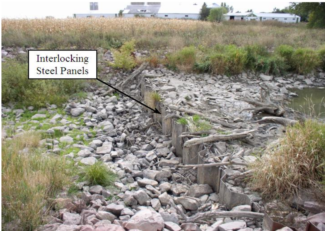
Figure 4.14. Installation of inter-locking steel panels to arrest channel erosion initiated by the construction of the by-pass channel between river miles 61.6 and 65.9.
