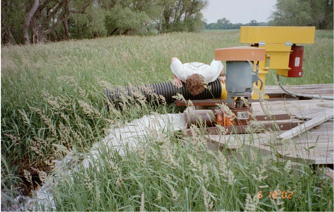
Figure 4.17. Discharge from sub-surface drainage collection tank near CoE cross-section #32 into SF LqP River.
