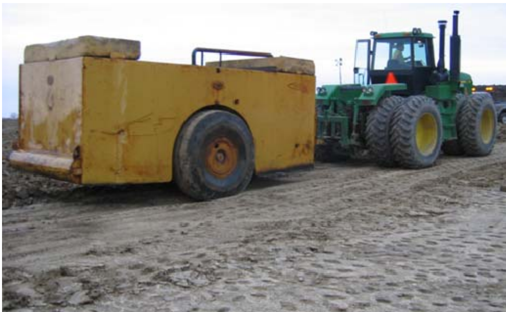
Figure 1.1. Test rolling at TH 212 construction site in Chaska, Minnesota on Oct. 5, 2006
