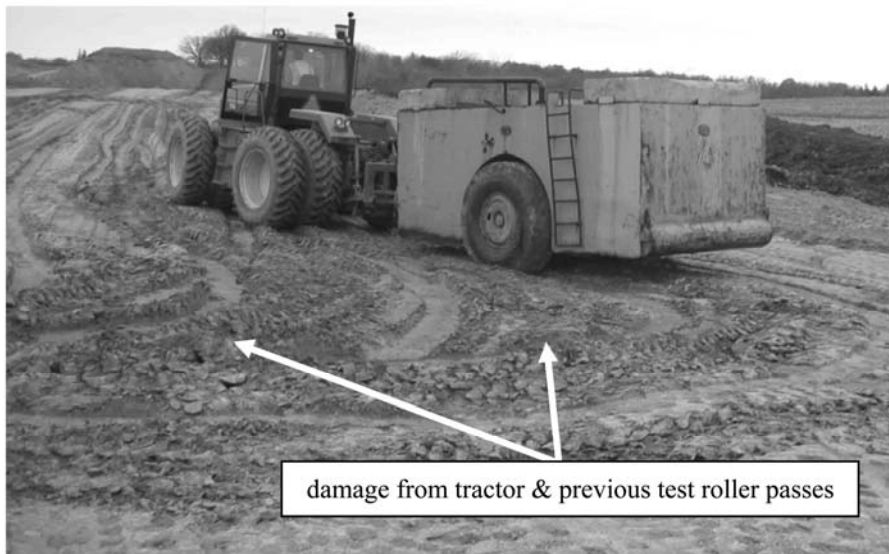
Figure 5.2. Damage to soil at field site with cohesive soil
