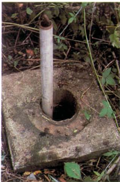
Improper well construction and abandonment.
