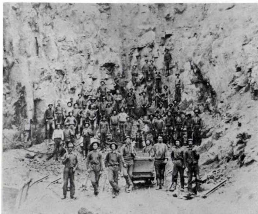
Picks and shovels were used in mining in the early days, when the Soudan was an open pit mine. Mine ore cars, drawn by mules, were used to haul the ore to the surface.
