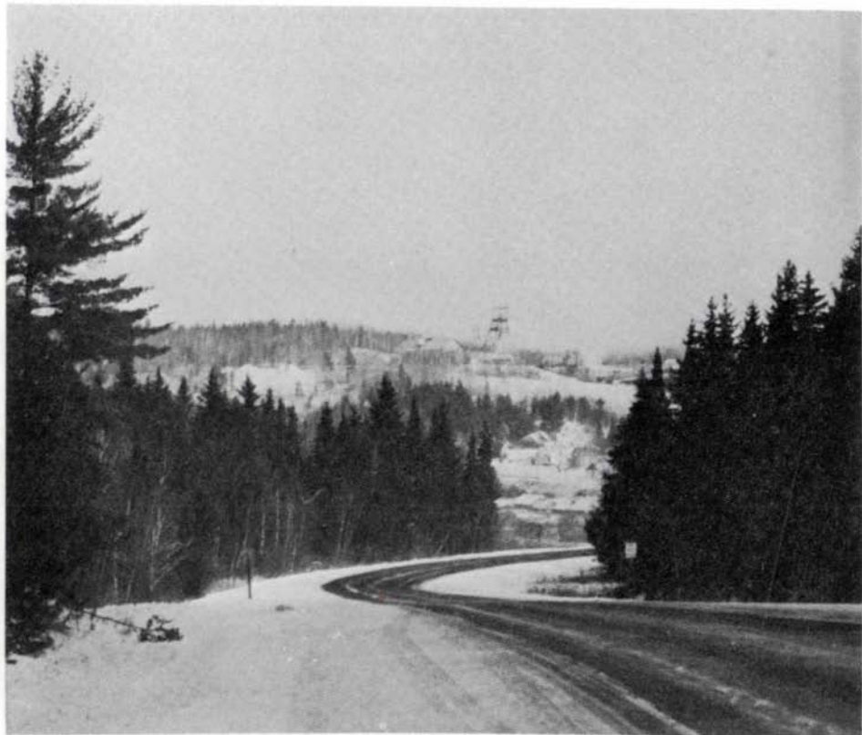
Soudan Mine, looking northeastward from State Highway 1. The head-frame visible in the distance is at No. 8 Shaft, which is used to take visitors underground.
