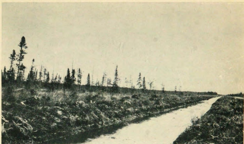
A. DRAINING A MUSKEG SWAMP IN ROSEAU COUNTY
