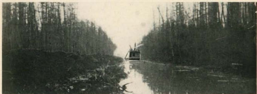
B. DREDGE EXCAVATING LARGE DITCH THROUGH A TAMARACK-PEAT SWAMP, BELTRAMI COUNTY PHOTO BY E. J. BOURGEOIS
