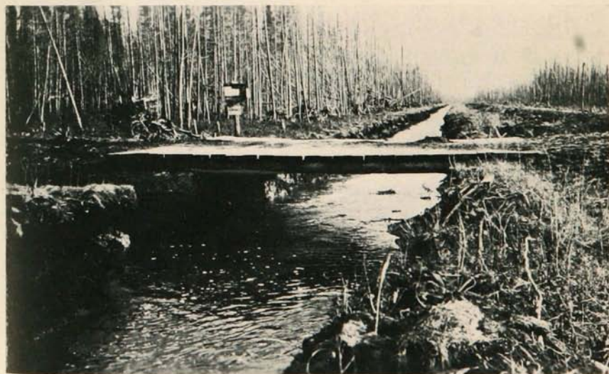
B. VIEW LOOKING ALONG DRAINAGE DITCH THROUGH A TYPICAL TAMARACK SWAMP WHICH HAS BEEN PARTLY BURNED. PEAT ABOUT 8 FEET DEEP. BELTRAMI COUNTY PHOTO BY E. J. BOURGEOIS
