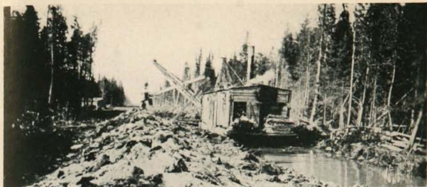
A. DITCH DREDGE AT WORK IN SPRUCE SWAMP, BELTRAMI COUNTY PHOTO BY E. J. BOURGEOIS
