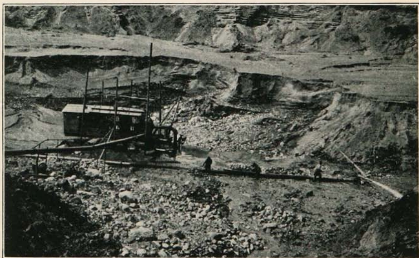
B. REMOVING OVERBURDEN BY HYDRAULIC METHOD AT THE HILLCREST MINE, NEAR IRONTON. SHOWS GIANT NOZZLE, CENTRIFUGAL PUMP, AND DISCHARGE PIPE PHOTO BY CARL ZAPFFE
