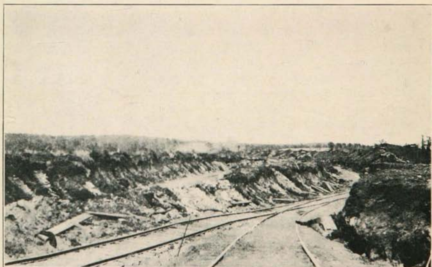
B. STARTING EXCAVATION WITH STEAM SHOVEL AT THE MAHNOMEN OPEN-PIT MINE, NEAR IRONTON PHOTO BY CARL ZAPFFE
