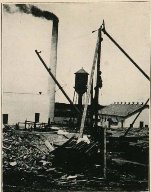
A. SINKING A CONCRETE SHAFT AT THE CROFT MINE, NEAR CROSBY PHOTO BY CARL ZAPFFE
