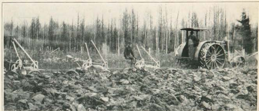
A. BREAKING GROUND AT MEADOWLANDS
