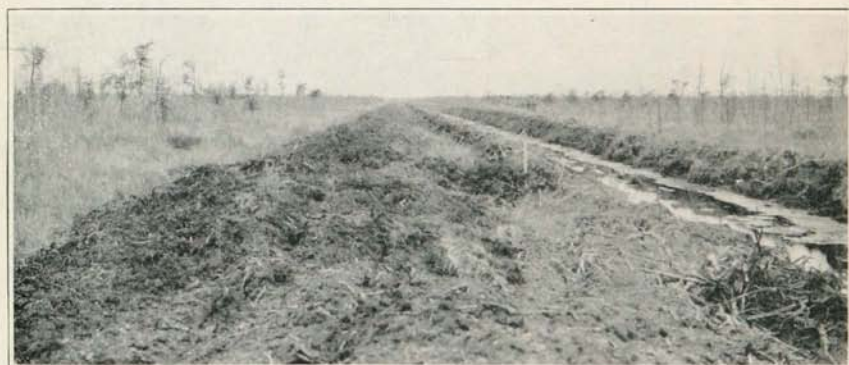
B. DITCHING A MUSKEG IN ST. LOUIS COUNTY
