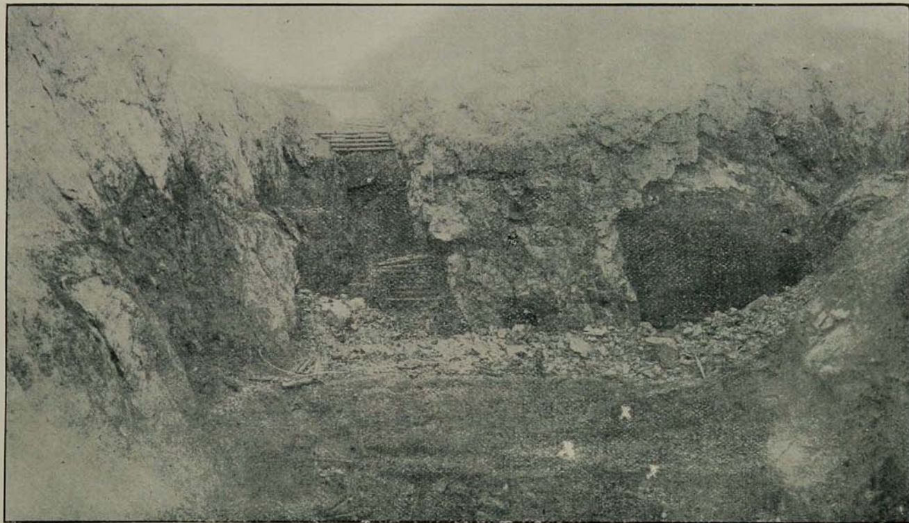
IRREGULAR VERTICAL TRANSITION OF THE JASPILYTE TO IRON ORE AS DEVELOPED IN THE STONE MINE, TOWER. (P. 63.)
