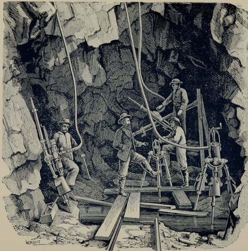
EXCAVATING FOR TUNNEL WITH INGERSOLL-SERGEANT ROCK DRILLS. P. 176.
