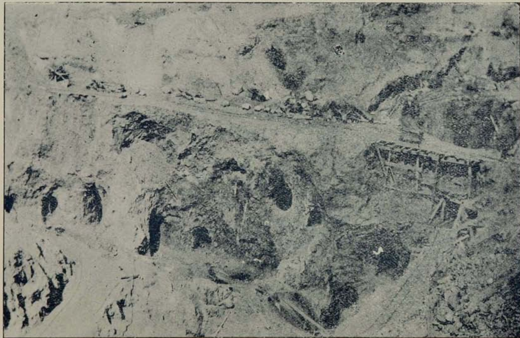
OPEN PIT OF THE CHANDLER MINE, ELY, SHOWING DRIFTS FROM WHICH ORE IS BEING TAKEN.
