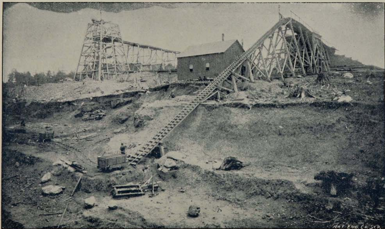
INCLINED HOIST FROM THE OPEN PIT, AND SHAFT TIMBERS FOR THE PERPENDICULAR HOIST. CHANDLER MINE ELY. (P. 167.)
