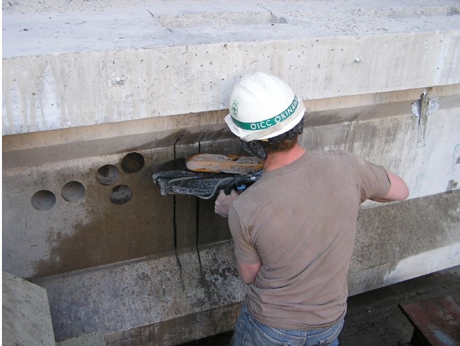
Figure C.3 Stirrup Removal
