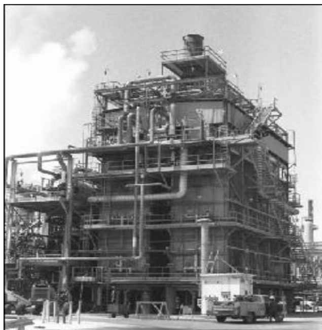
Figure 1.3: A commercial steam cracker requires contact times on the order of \tau \approx 1 second. The millisecond reaction time of CPO means that this plant can be scaled to approximately the size of the truck parked in front. Photo from [36]
